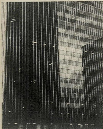
For lights of regular shape (rectangular or square) and less than 200 sq in. in area, tinted clean-cut edges will suffice.
