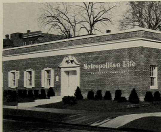
SPRINGFIELD, MASSACHUSETTS: 5,000 sq. ft. Metropolitan Life Insurance Company branch office building. Contractor: A. C. Dufault. (Design by Metropolitan Life Insurance Company architects.)
