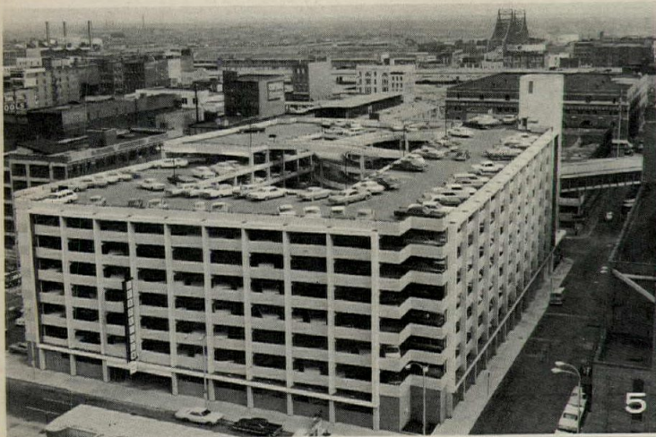
5. Parking Structure for Stix, Baer & Fuller Dept. Store, St. Louis— Post-tensioned beams make long clear-spans more practical and economical. Architect-Engineer: Enco Associates, Inc. Parking Consultants: Richard C. Rich and Associates, Inc. General Contractor: G. L. Tarlton Contracting Company.
