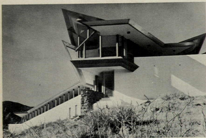
Residence for Dr. Robert Willard, Boulder, Colorado. Architect: Charles A. Haertling.
