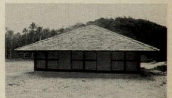
Simple detail and careful design produced houses for $14,000 each, half usual government house cost.
