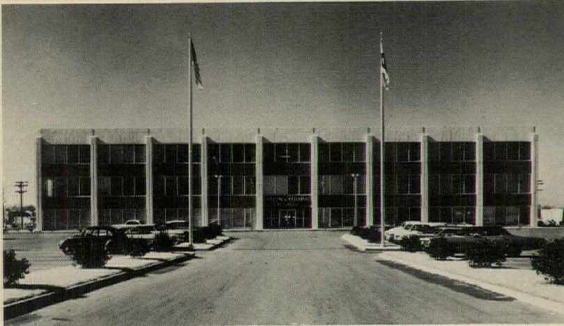
ALLEN & O'HARA BUILDING, Memphis, Tennessee. Architects: Robert Lee Hall Associates, Inc. General Contractor: Allen & O'Hara, Inc. Three Dover Oildraulic Elevators installed by Dover Elevator Co.
