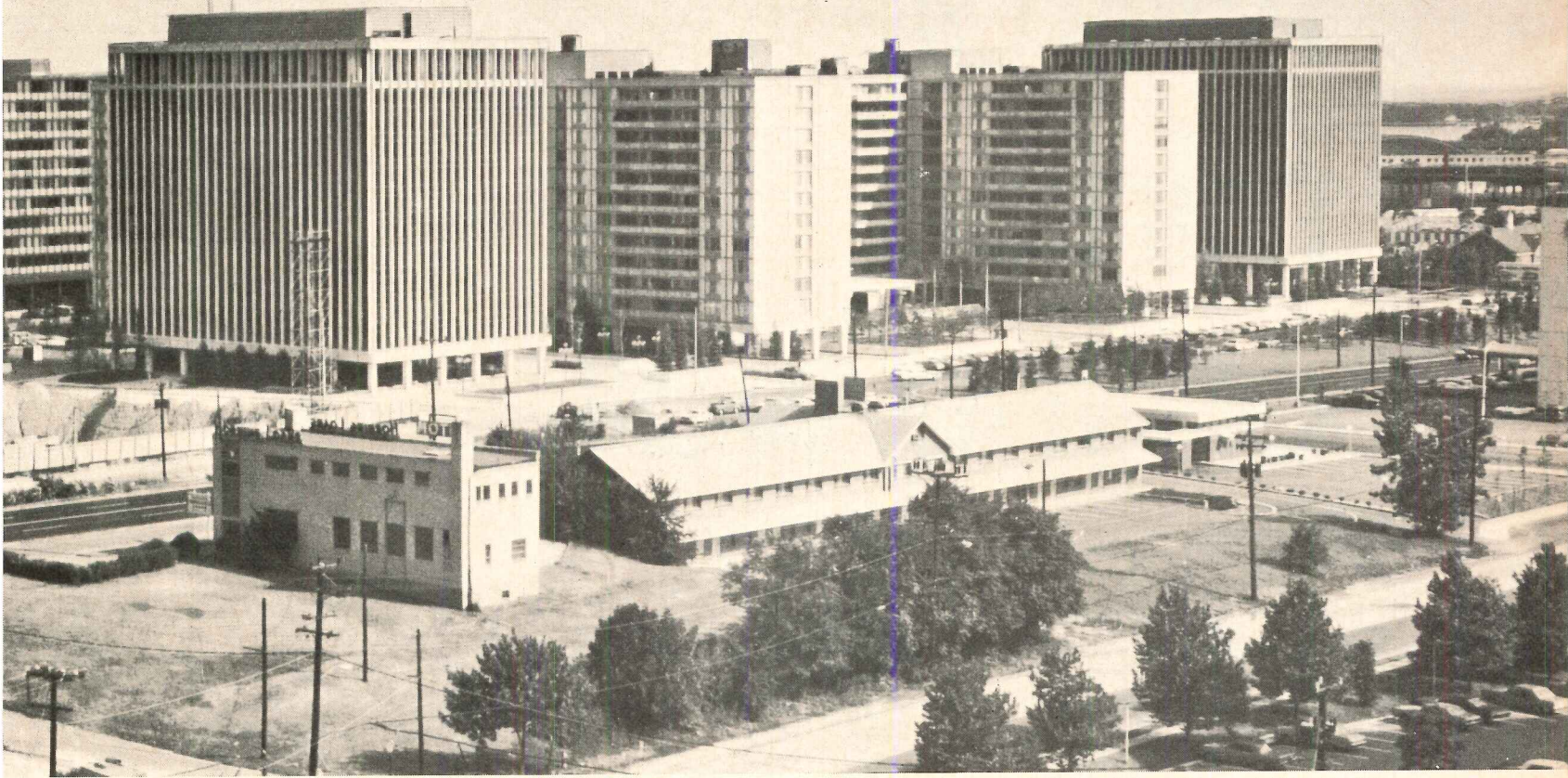
Ceco Steelform Service for 790,000 sq ft of monolithic concrete joist construction 12,700 tons of Ceco-fabricated Reinforcing Steel 480,000 sq ft of Cecocolor Anodized Aluminum Windows and Curtainwalls
