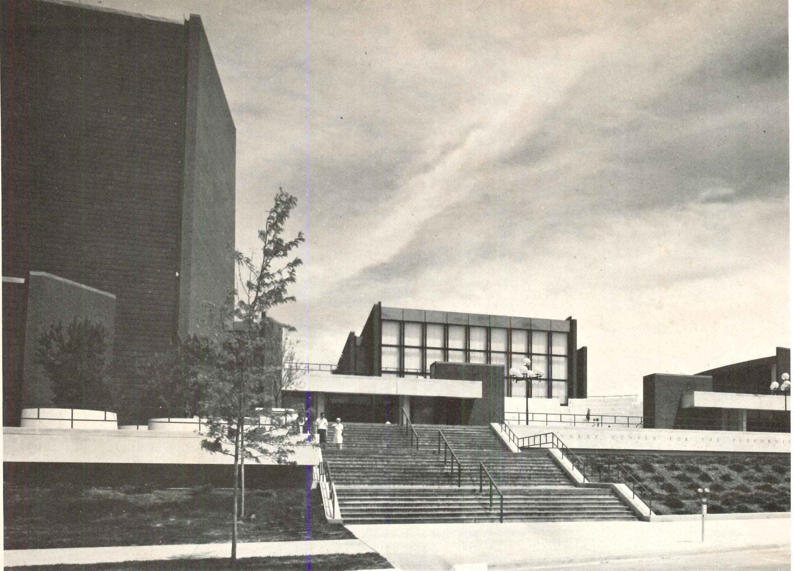
FIVE SINGLE-PURPOSE THEATERS CONNECTED BENEATH A PODIUM: KRANNERT CENTER FOR THE PERFORMING ARTS
