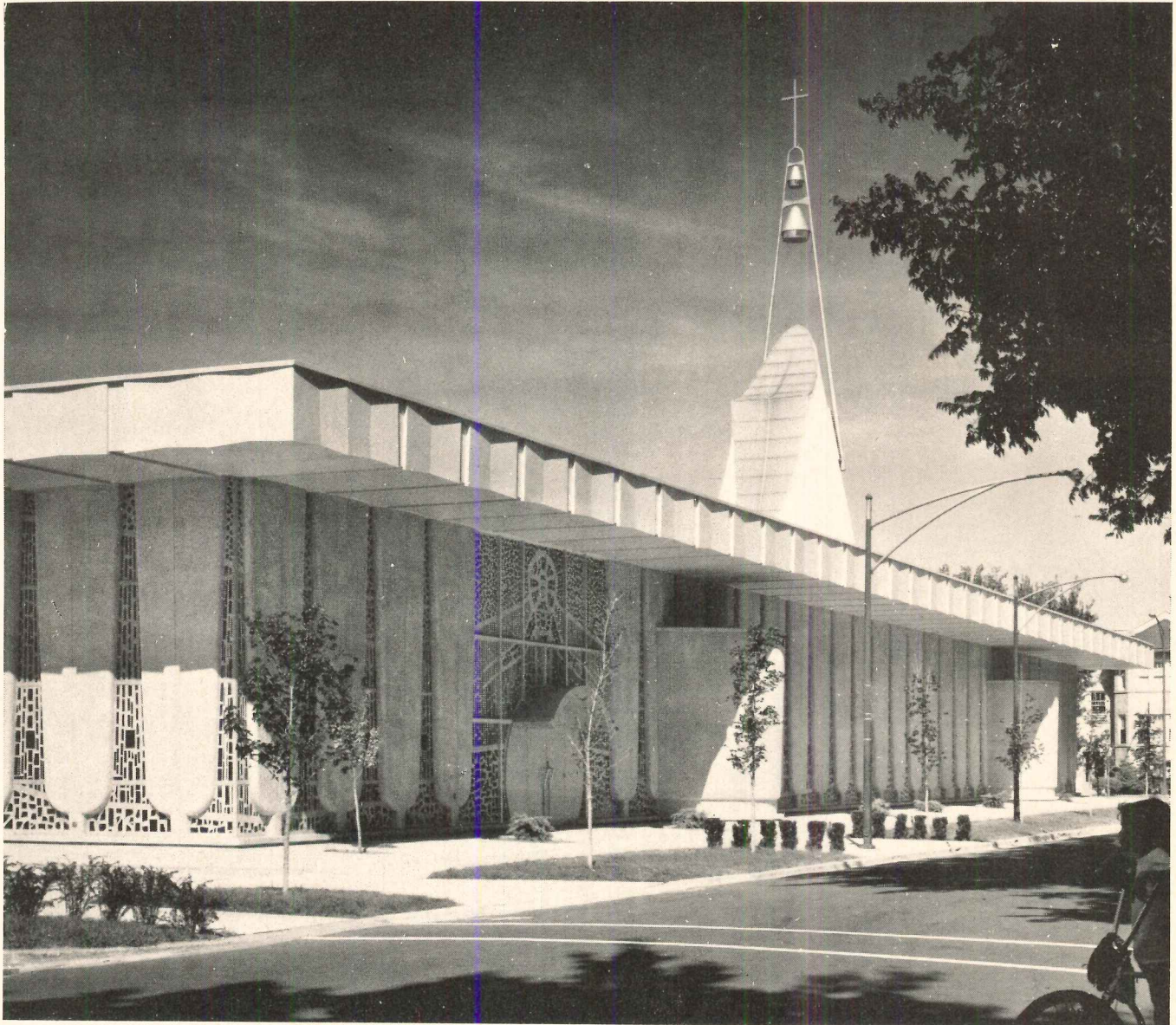
CREDITS: St. John Bosco Church, Chicago; Architect: Belli & Belli, Chicago; General Contractor: Chell & Anderson, Inc., Chicago; Lathing and Plastering Contractor: William A. Duguid Company, Chicago
