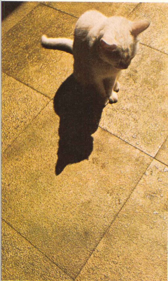
Bronze floor tiles (left). Pebble textured bronze on copper sheet applied directly to concrete or plywood. Needs only minimum care. Foot traffic adds varied highlights of muted gold tones.
