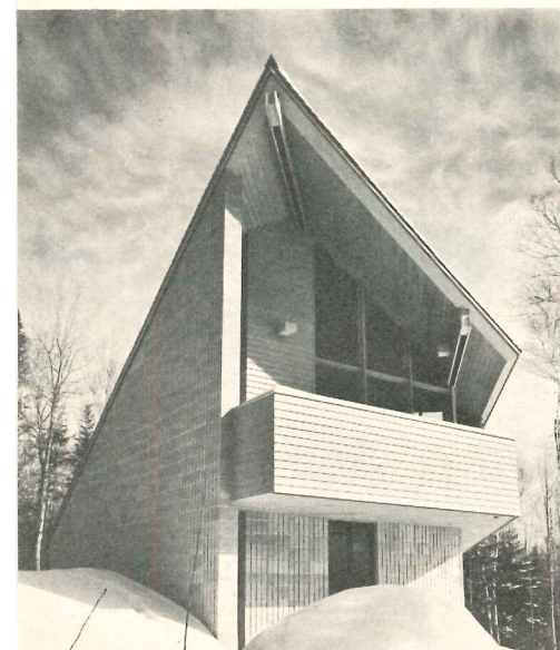
The logical combination of masonry and frame construction gives a crisp clarity to the house (below) and the sheltering roof appears to float above the band of south-facing windows. The massive chimney not only stabilizes the structure but provides a suitably-scaled fireplace. From the built-in couch, skiers can watch the sun set on distant peaks.
