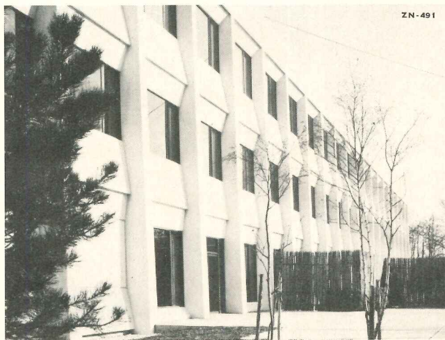
IBM's beautiful Data Processing headquarters utilizes galvanized re-rod to prevent sub-surface rust and consequent staining.
