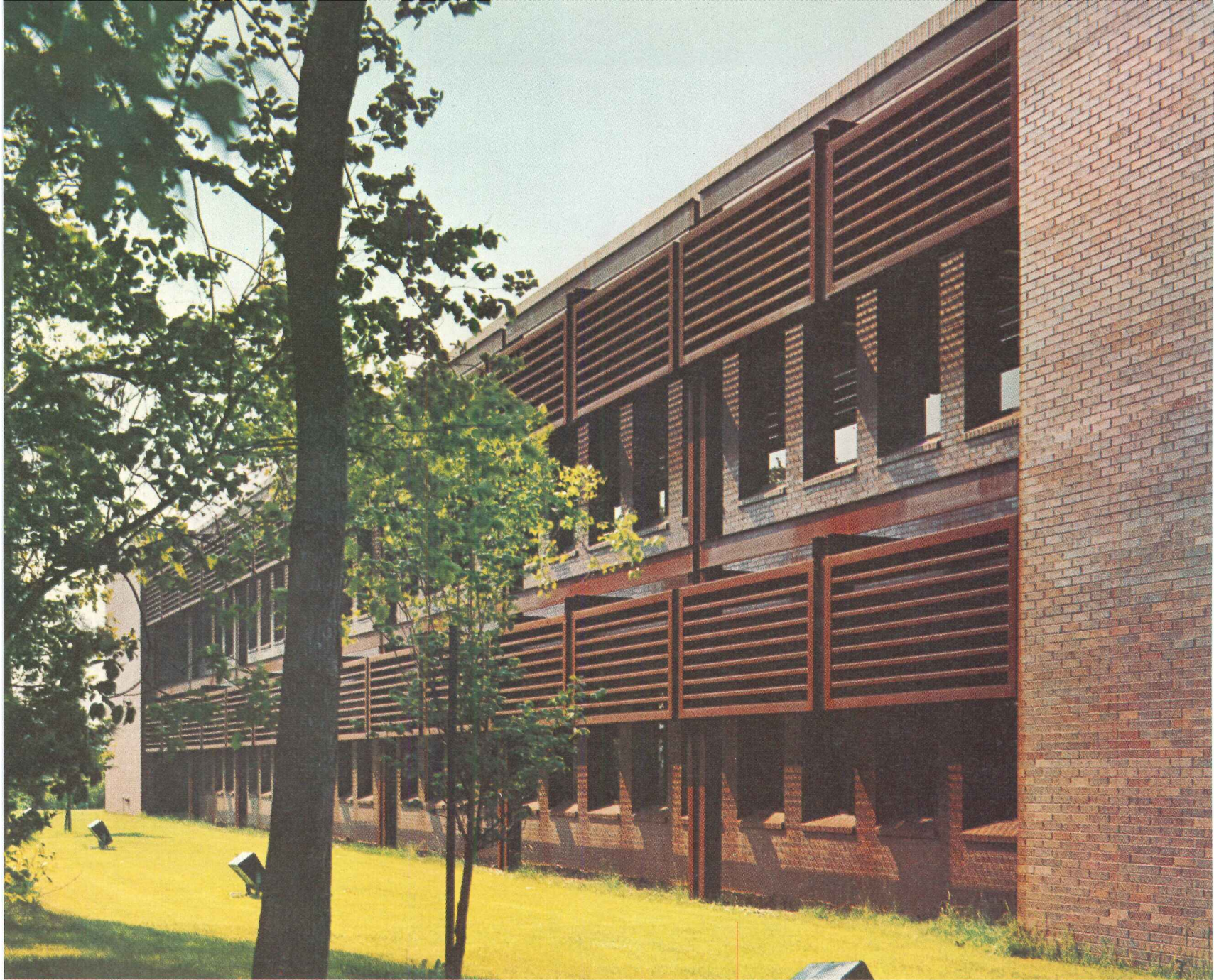
Owner: Itek Corporation; Architect-Engineer: Neal Mitchell Associates Incorporated; Fabricator and Erector: Novel Iron Works, Inc.; General Contractor: Lewis C. Bowers, Inc.
