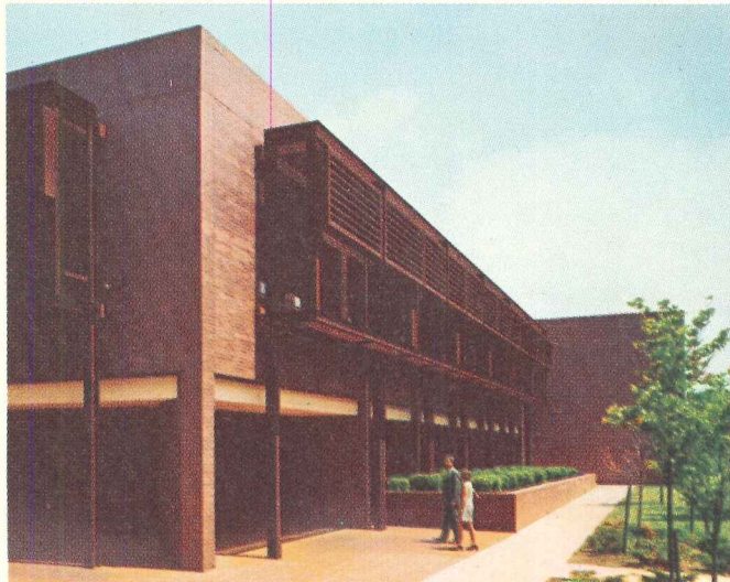
Main office entrance. Loose bricks, placed in sand around base of Weathering Steel columns to catch oxidized run-off, will be replaced and mortared after the steel matures.
