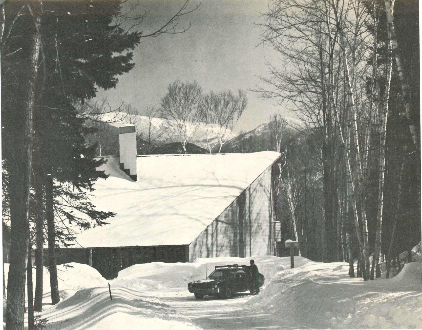
The logical combination of masonry and frame construction gives a crisp clarity to the house (below) and the sheltering roof appears to float above the band of south-facing windows. The massive chimney not only stabilizes the structure but provides a suitably-scaled fireplace. From the built-in couch, skiers can watch the sun set on distant peaks.
