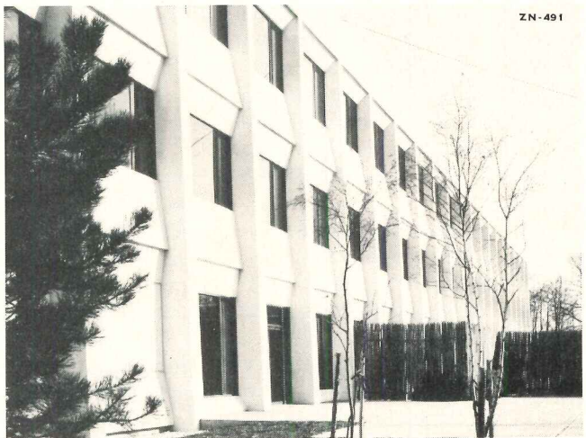
IBM's beautiful Data Processing headquarters utilizes galvanized re-rod to prevent sub-surface rust and consequent staining.
