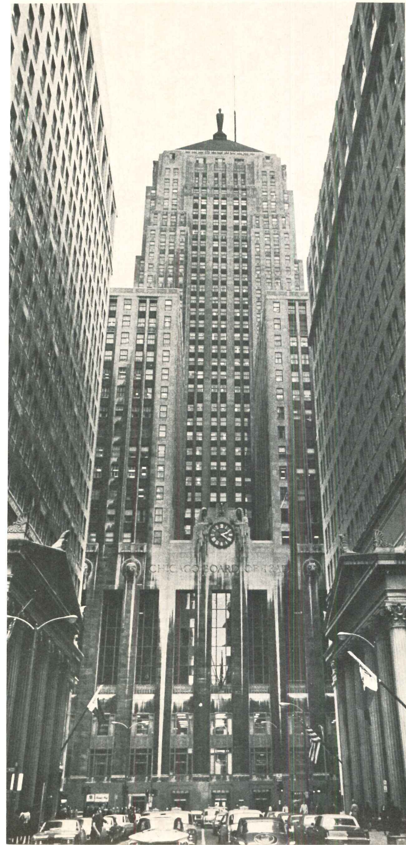
Chicago's Board of Trade building: preservation and renovation
