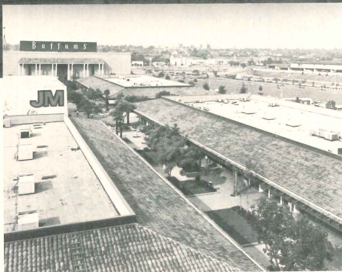
Fashion Square Shopping Center, La Habra, California, an open air mall. Lennox roof mounted heat pumps provided an ideal design solution in Southern California's mild climate. Owner: U.I.D.C., Inc. Architect: Welton Beckett & Associates, Los Angeles.
