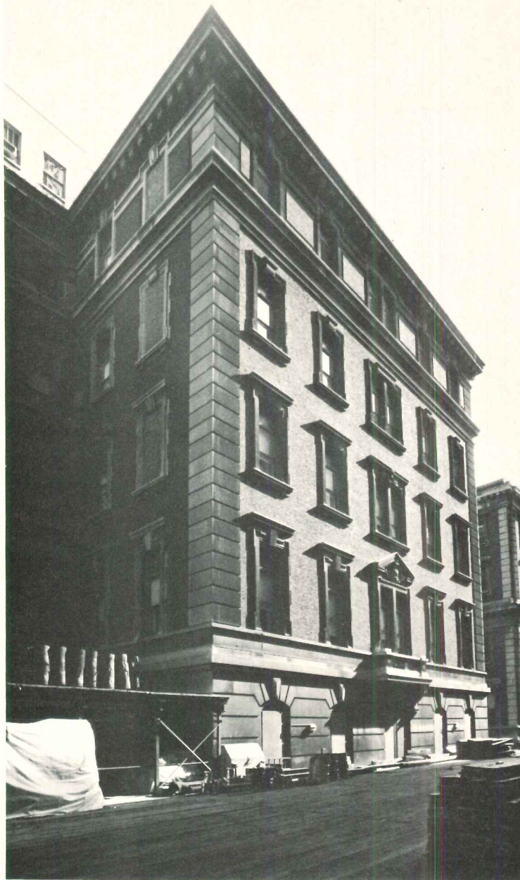
Above is the facade of the old open-ward unit which has been allowed to remain intact, with some changes in elevation and circulation at the ground level. Before, during, and after stages of reconstruction are shown from top to bottom in the series of three photographs at the right, and the section, far right, illustrates construction of the interstitial mechanical spaces.
