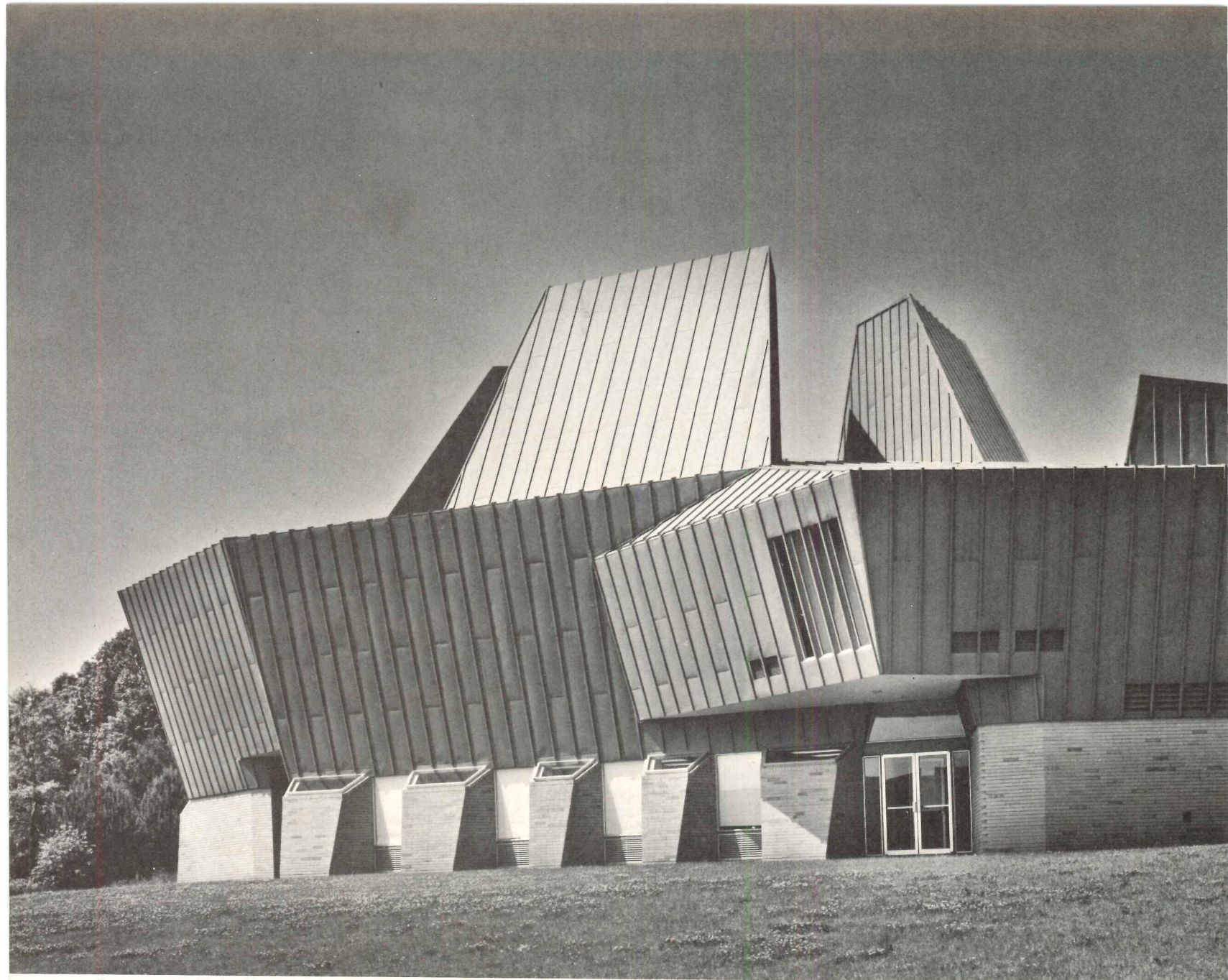
Congregation Beth El, New London, Conn.; Architect: Paul Rudolph, FAIA, New York, N.Y.; Roofer: H. R. Hillery Company, Groton, Conn.
