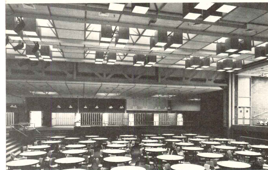
The wide variety of lighting is apparent by examining a classroom area (top), the industrial arts wing (center), and the dining commons (above). The lighting plan, right, covers the width of one 25-ft structural bay, and, in length, goes from an illuminated exterior wall, across the mezzanine, and across the Instructional Materials Center. Lighting in the dining commons is incandescent lamps set in the wooden-cube fixtures. Industrial arts and art wings have fluorescent panels.
