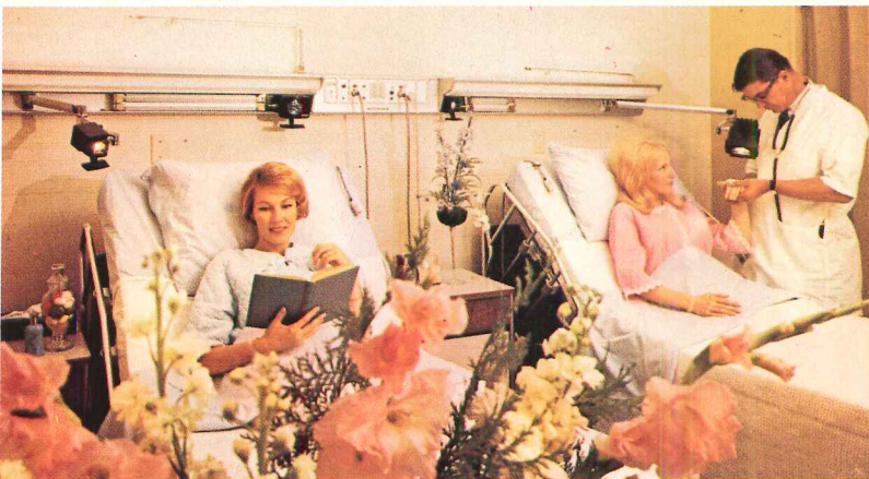
One example of Keene hospital lighting is this console containing fluorescent fixtures, plus examination and reading lamps.
