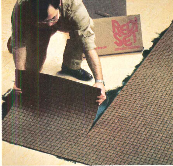
lay the pregrouted sheets,
