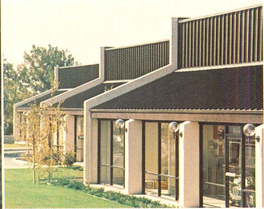
The system permits pleasing roof variety.
