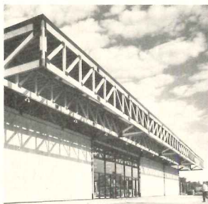
Cover: Nagle Lumber Company Iowa City, Iowa Architects: Booth and Nagle Photographer: Philip Turner
