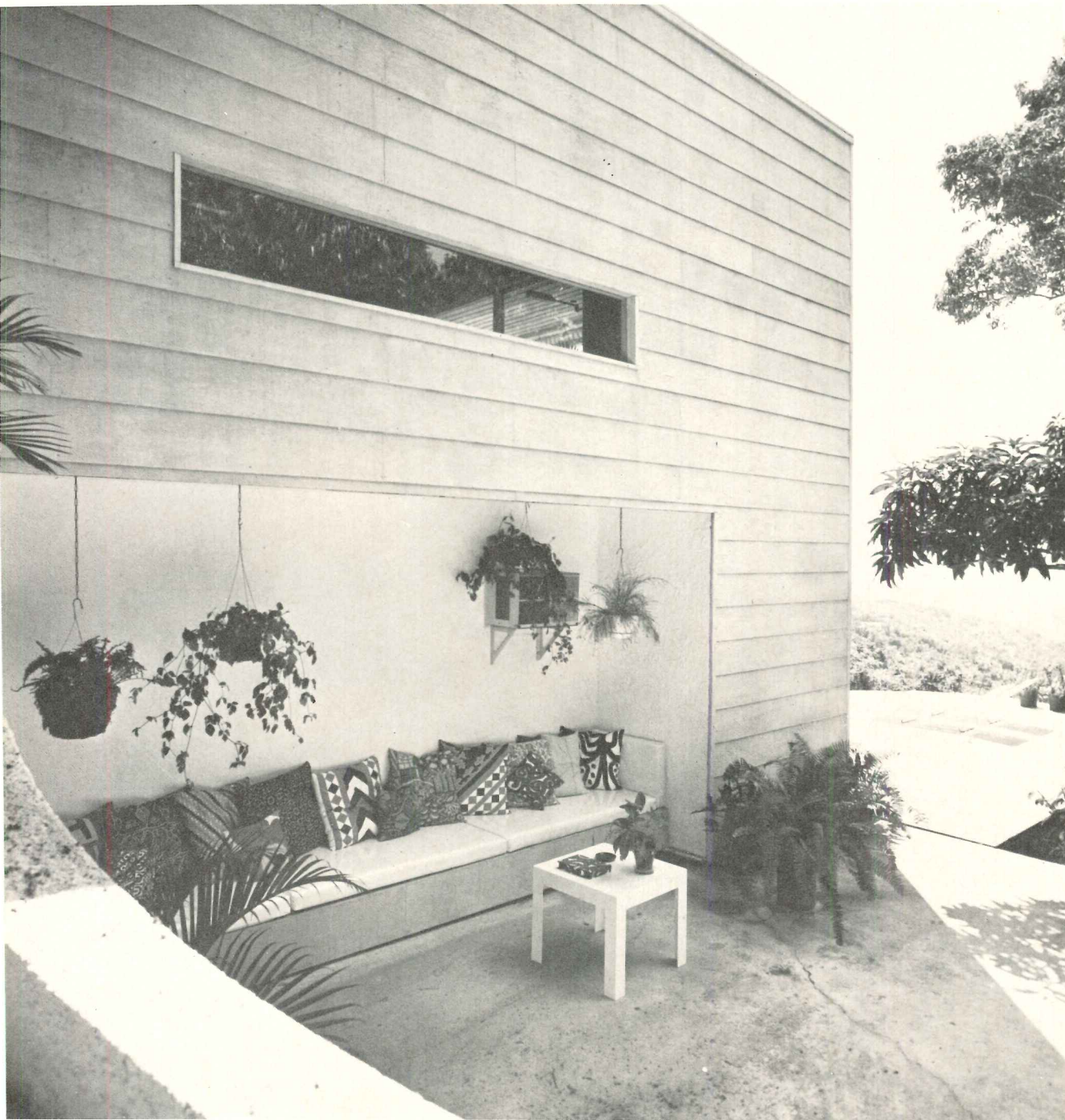
On the north side of the house, at right angles to the direction of the slope, Bates has developed a small terrace protected from the sun. The master bedroom (photo right) with a strip window over the headboard, overlooks the terrace and opens, at the side, into a covered gallery.
