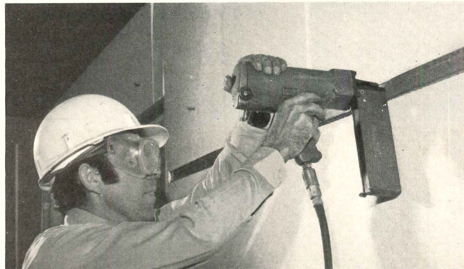
Nail through Foam to masonry.
