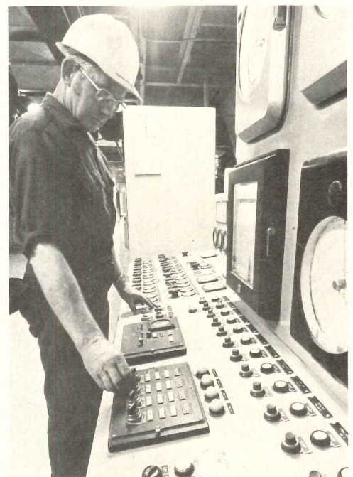
Steam plant is just a half-mile away.
