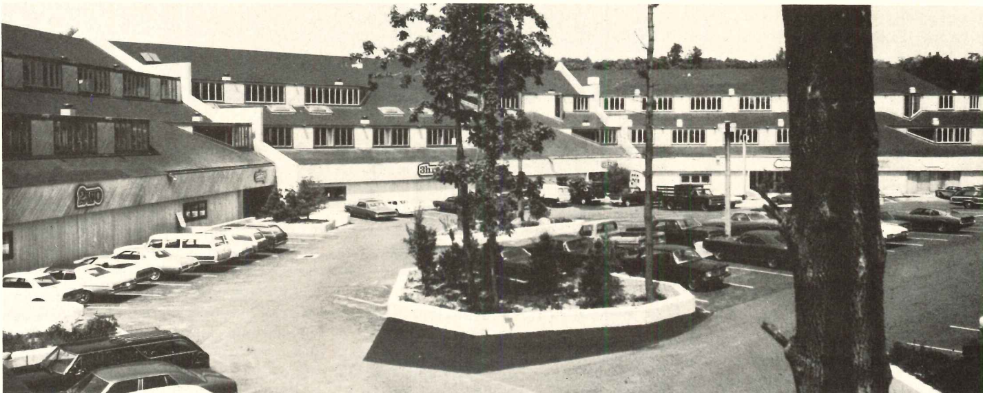
Sloping roof of The Exchange mall helps building appear small in scale despite its four levels and ¼-million square feet.
