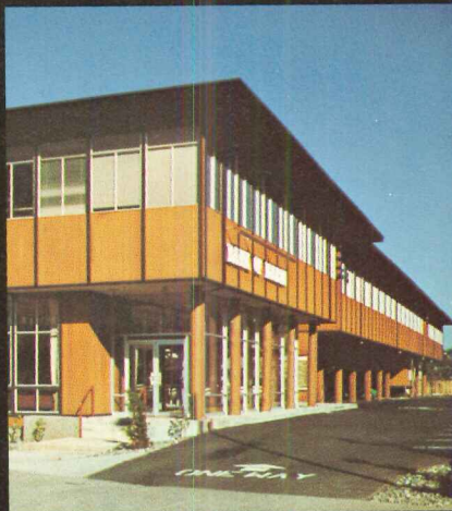
Office Building—Sausalito, California Arch.: Wurster, Bernardi and Emmons, Inc., AIA Structural Engineer: W. B. Clausen
