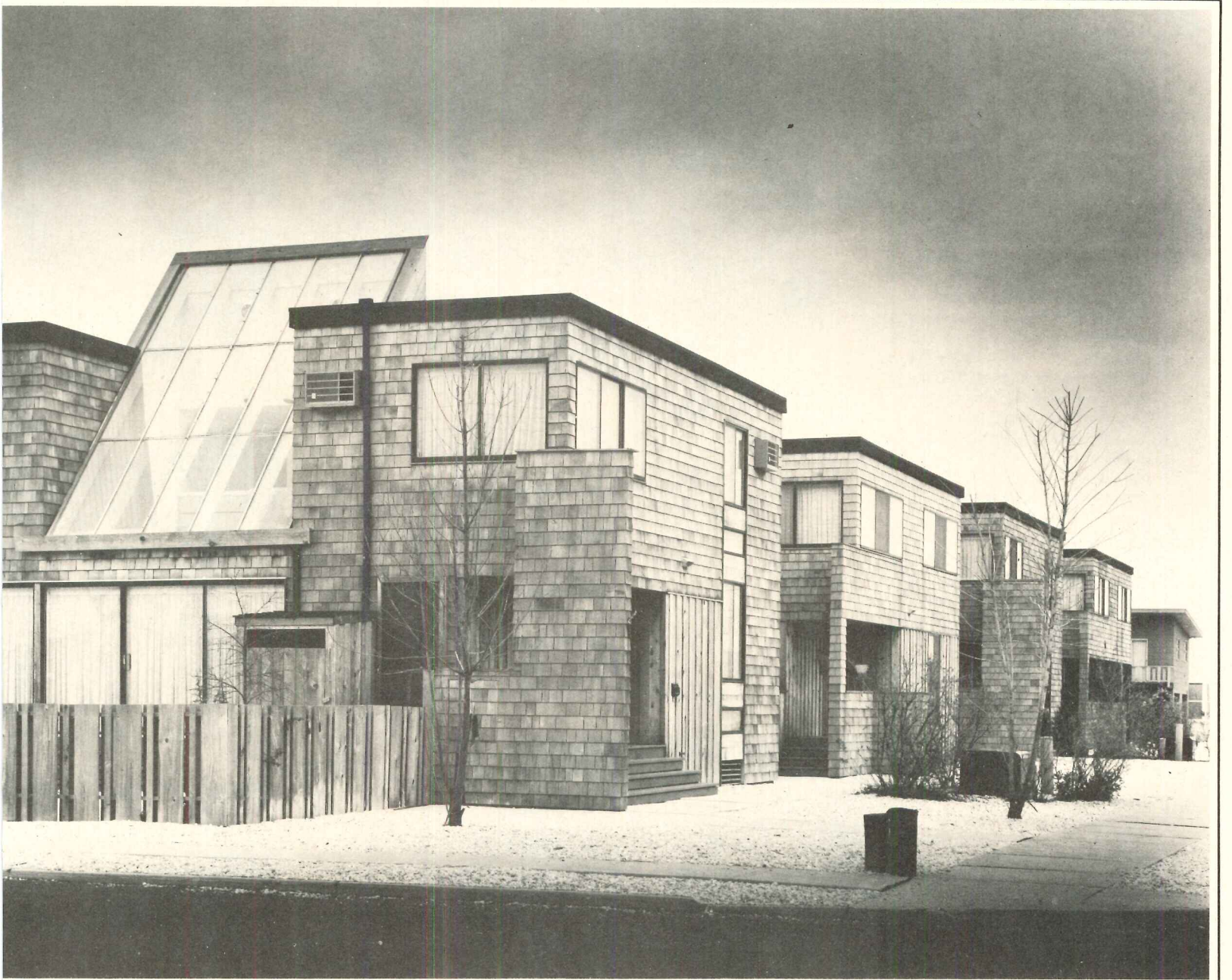
Working with the side yard restriction, Sauer provided each apartment with one blind outside wall (see plan), a design device that protects the privacy of each individual side yard.
