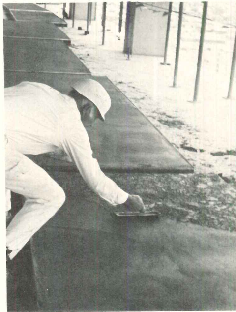
On-slab fabrication of the cement-plaster panels for the Hyatt Regency in Phoenix is shown above. With the mobility afforded by open floor space, it was possible for fabrication to proceed rapidly. Scratch coat has been applied in the photo above, left, and the finish coat is shown above, right.
