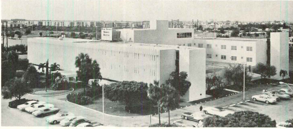
Palm Springs General Hospital, Hialeah, Florida, four floors, masonry construction, 250 beds
