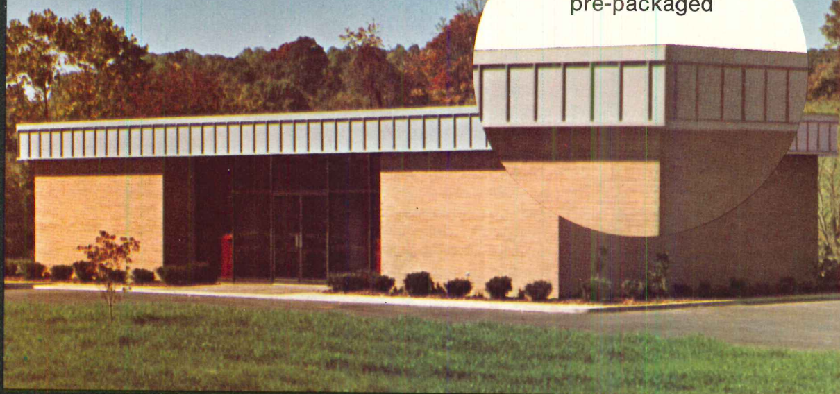
Greene County Bank, Greenville, Tenn., Architect: Boyd & Arthur, Roofer: Hicks Sheet Metal Co.
