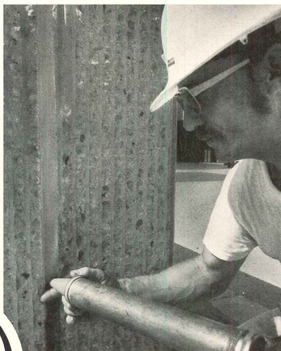
Applying an LP® polysulfide-base sealant.
