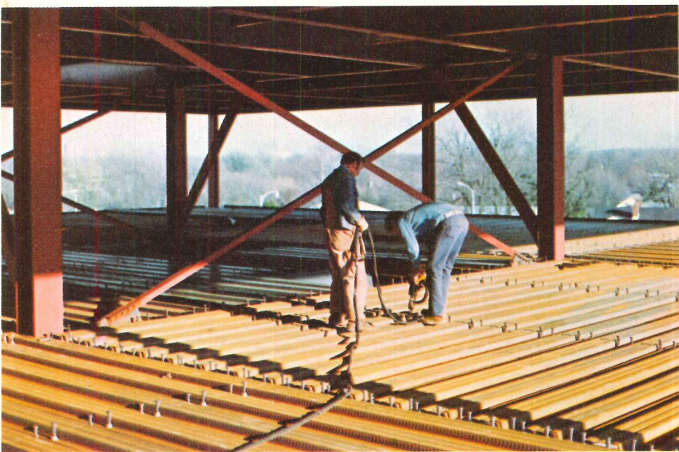
The floor system consists of a 3/4-in. lightweight composite concrete topping over 2-in. non-cellular composite steel deck. Floor-to-floor height is 12 ft. Bethlehem furnished all of the structural steel requirements for the building.
