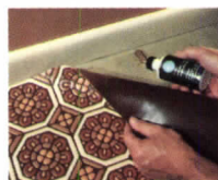
Tredway installs over concrete with just a band of adhesive.
