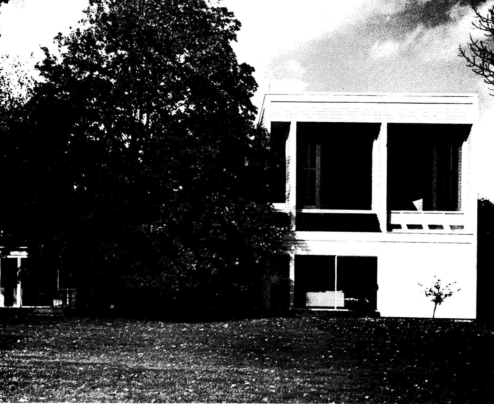
The large openings on the upper level of the new addition are recessed to control the sunlight admitted. Further control is provided by 3- by 10-foot operable sunscreens (photos above and at right).
