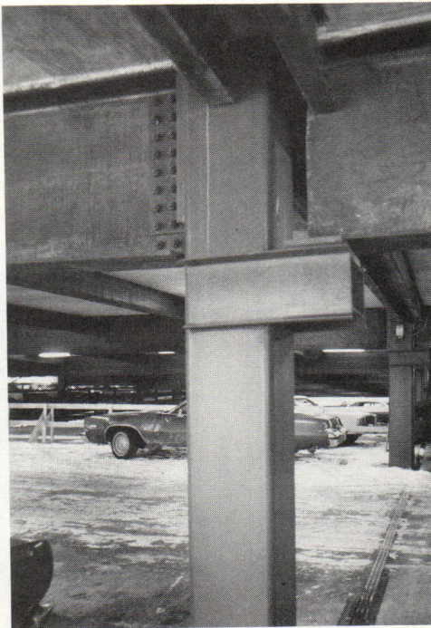
Below: thermal expansion of girders is provided for by sliding joint comprised of bracket and Teflon pad.
