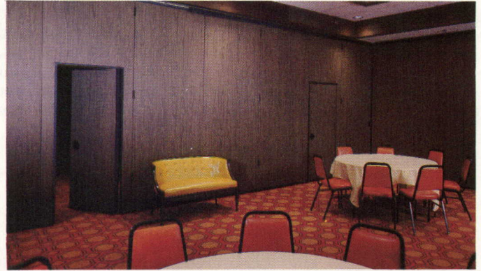
Passdoors can be built into the panel for room-to-room access. Panels stack neatly in storage pockets when not in use.
