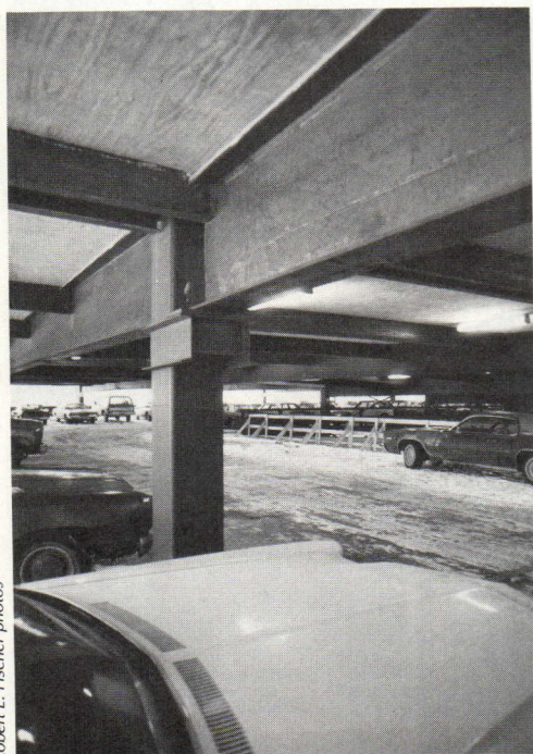
Below: thermal expansion of girders is provided for by sliding joint comprised of bracket and Teflon pad.
