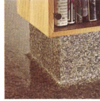
Coving like this helps eliminate corners where dirt can hide.
