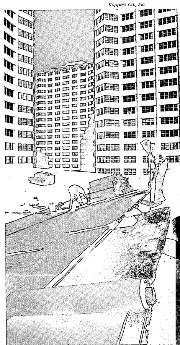
In a reroofing application, workmen laid a bitumen-based composite membrane on the roof over the lobby of the Hotel Intercontinental Miami. The aluminum top face protects the membrane from the sun's rays. Roofing consultant was Peter Corsell Associates.
