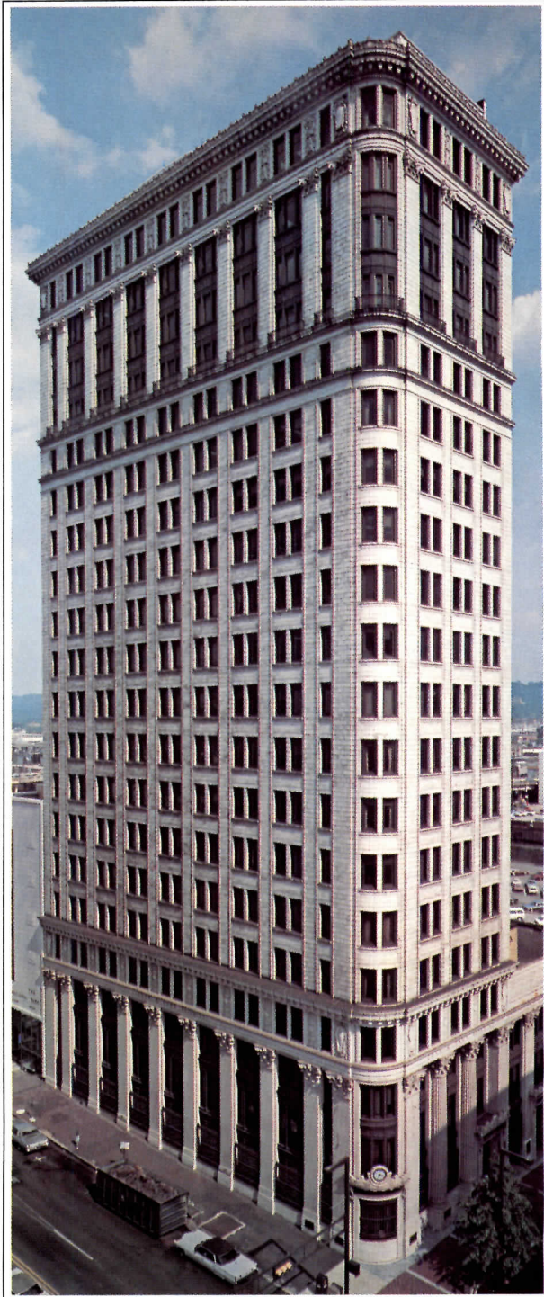
John A. Hand Branch Office, First National Bank of Birmingham, Alabama's Largest Bank. Brice Building Co., Inc., General Contractors.
