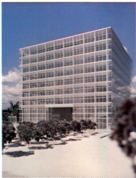
• Owner, Engineer and Architect: Marvin W. Voelker, VP, Hooker Niagara Office Corp., Niagara Falls, N.Y., Alan M. H. Sloan, VP, Engineering and Mark R. Mendell, AIA, Sr. VP, Cannon Design Inc., Grand Island, N.Y.
