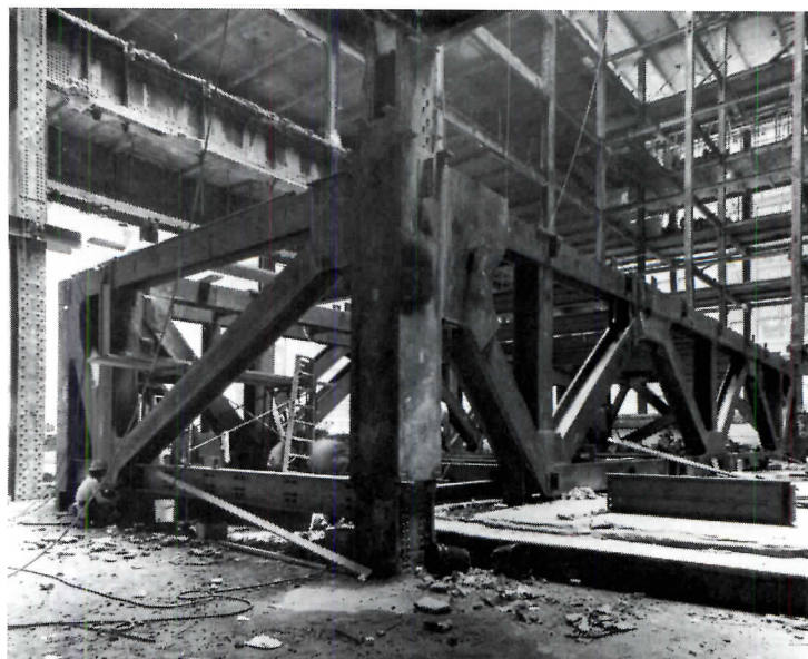
A workman, in the lower left foreground, lends scale to the trusses. The transfer structure is 12 ft deep, 36 ft wide and spans 73 ft across the most westward arrival area of Grand Central Terminal (under the Biltmore).
