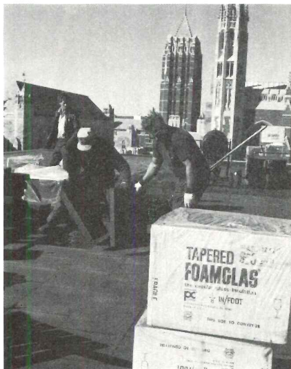
Tapered FOAMGLAS® Roof Insulation Systems drain water off the roof quickly and eliminate ponding.
