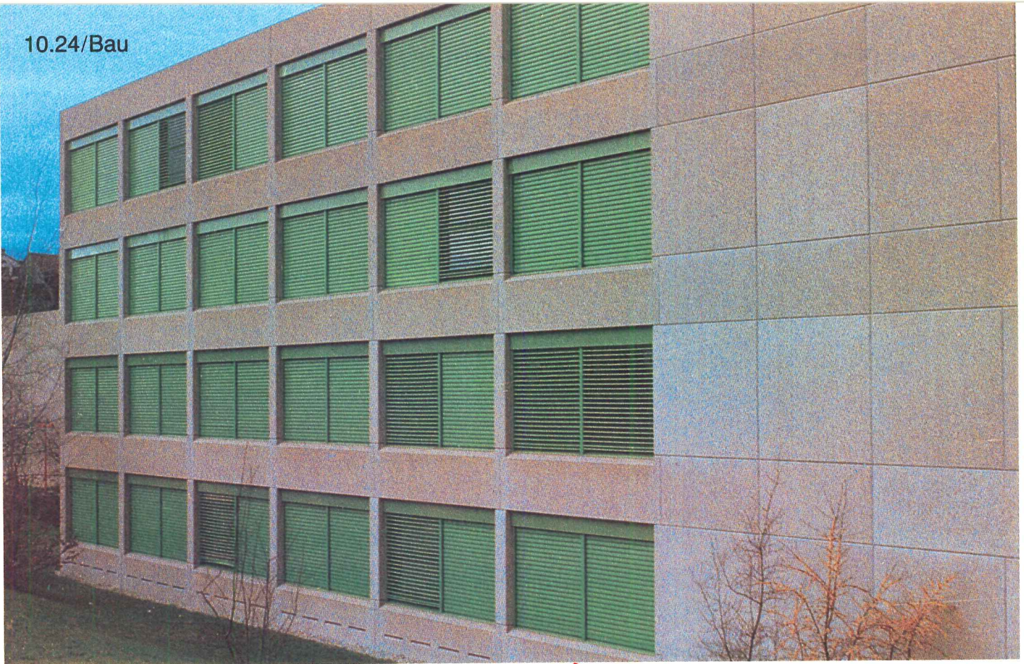
Above, weekend overtime workers in various offices use local override controls to open own blinds to enjoy natural daylighting.
