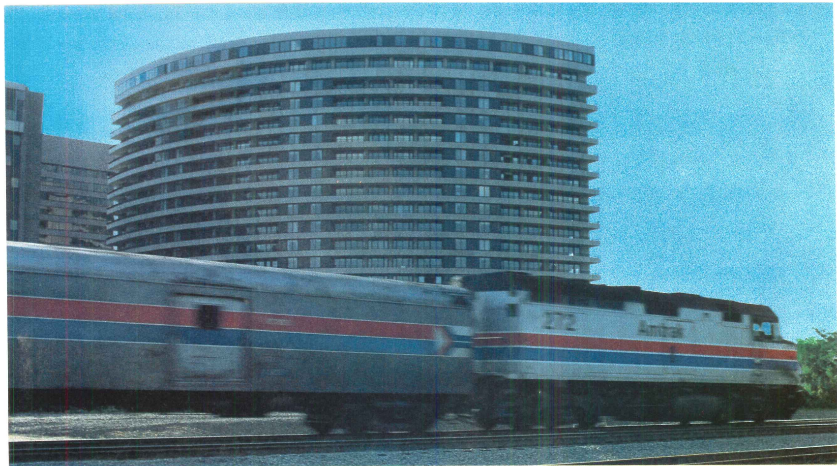
Washington D.C.'s Crystal City residential and commercial complex was designed by Weihe, Black, Jeffries, Strassman & Dove of Washington D.C., and is managed by Charles E. Smith Building Corporation
