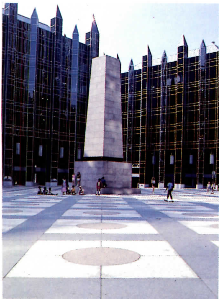
At close range, the curtain wall's chameleon-like character displays a rich array of surface qualities, intensified by self-reflection. Not only do separate buildings mirror each other, parts of individual buildings reflect themselves. For example, corners are doubly spliced with aluminum mullions and their reflections (right).
