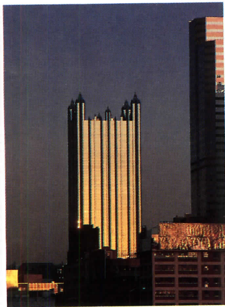
Like other reflective glass curtain-wall buildings, PPG Place visually responds to the varying ambient light of dawn, dusk, night, and full sun. Unlike other glass towers, PPG's "pleats" significantly extend its vocabulary of surface effects. At times, the Tower's monolithic form on the urban skyline is turned into a bundle of delicate, radiant shafts.
