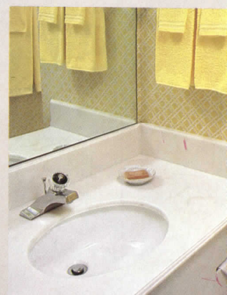
Formal edge treatment adds to appeal of guest bath in Amway Grand Plaza Hotel, Grand Rapids. DeWinter Associates, Inc., architects.
