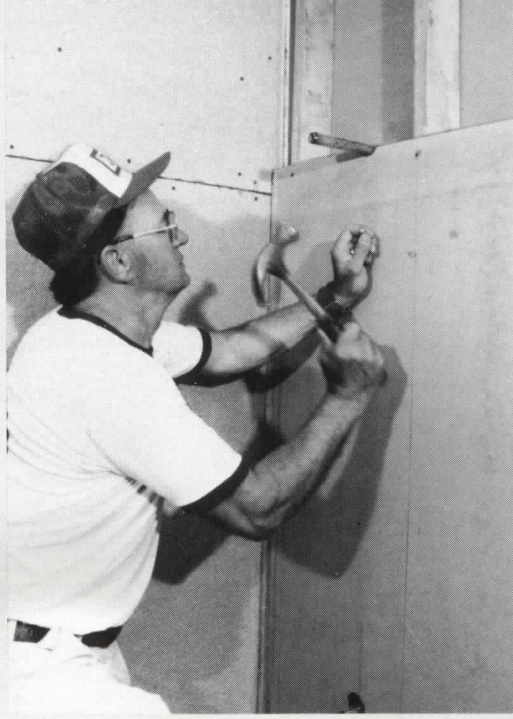
NEW BEST WAY: Same kind of strong, water-resistant performance, now in quickly-installed cement panels.
