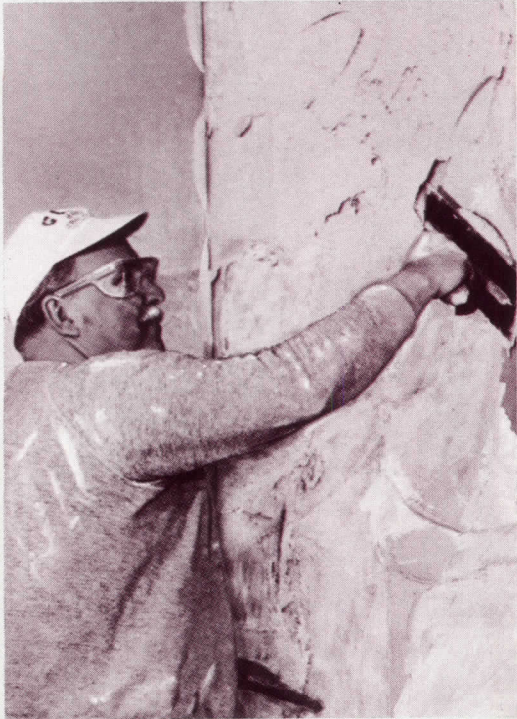
BEST WAY: Portland cement mortar over lath was great when labor costs and time delays were acceptable.
