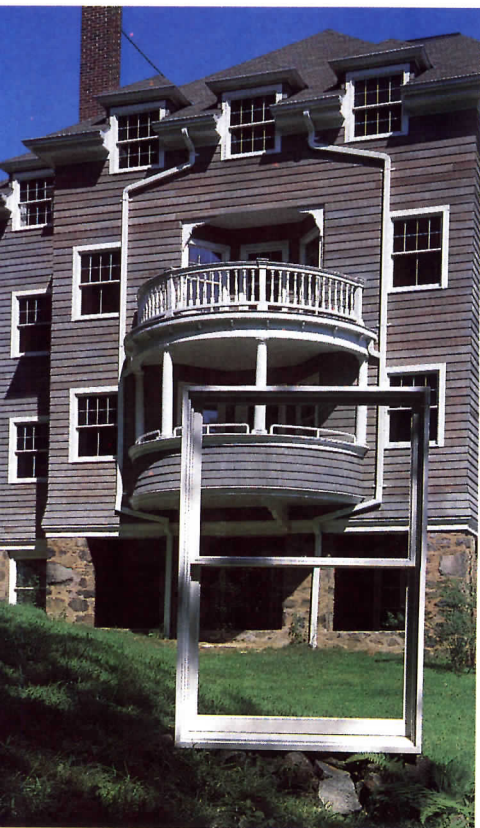
Simpson Hall Nyack College South Nyack, New York Architect: Schofield/Colgan Architects Nyack, New York Single vertical grilles not by Andersen.
