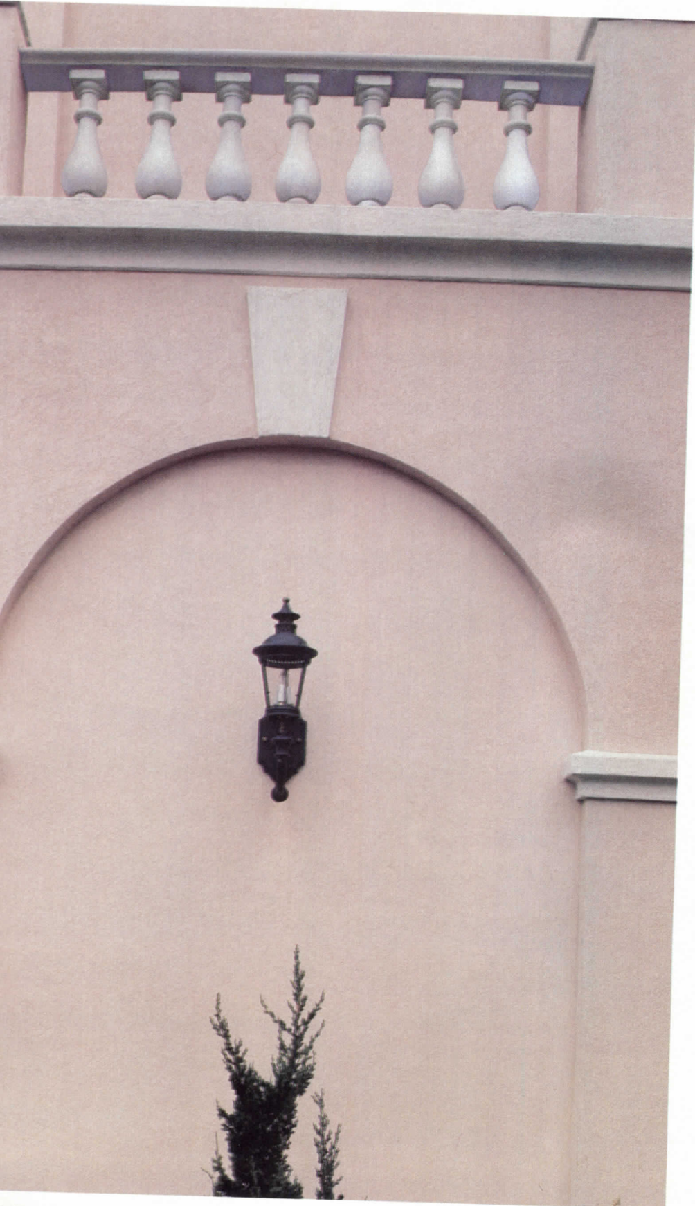
Highlawn Pavillion, New Jersey
