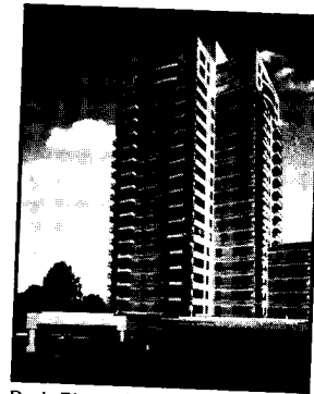
Park Plaza Condominiums Wilmington, Delaware Salkin Group, Inc.
