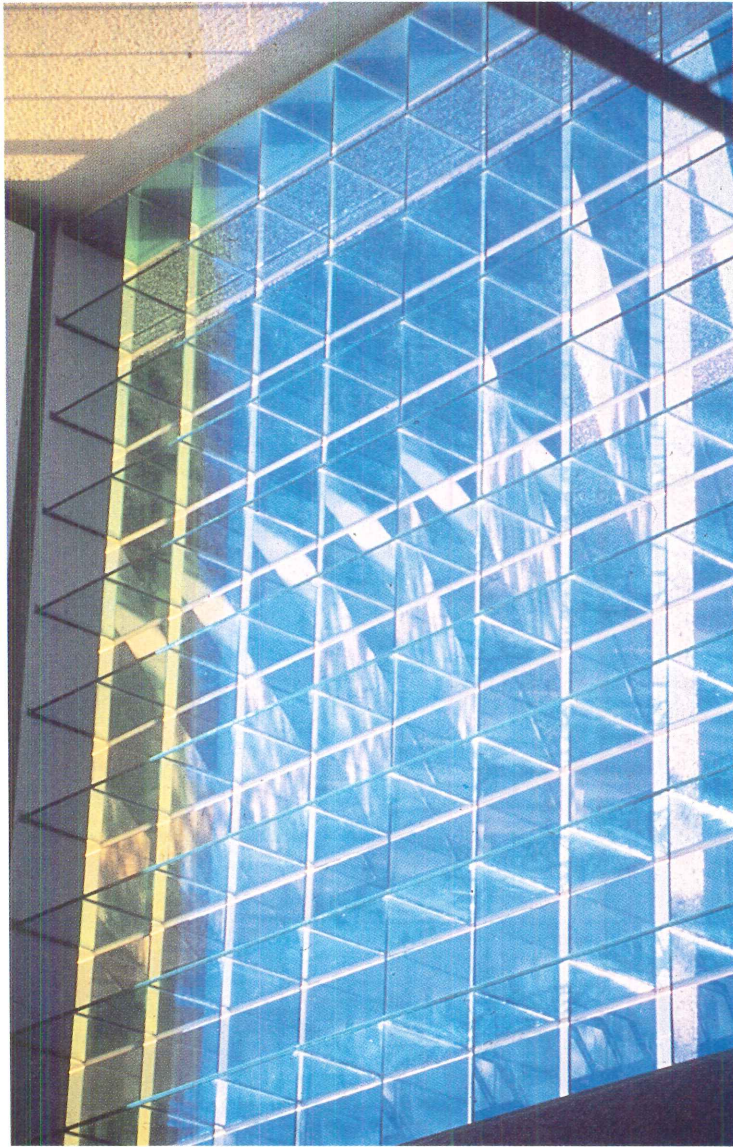
The window above was created by James Carpenter for the Christian Theological Seminary chapel in Indianapolis. Carpenter's commission came from the architects for the chapel, Edward Larrabee Barnes/John M. Y. Lee, P. C., Architects. The structurally glazed and gridded glass has a dichromic coating on its horizontal members. The coating works like a prism, reflecting and transmitting a complex pattern of colored light that changes in conjunction with the position of the sun—the light is meant to be spiritual and ephemeral.
