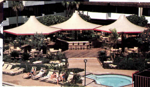
Clustered tension membrane Modular Shelters, Pompano Beach, Florida.
