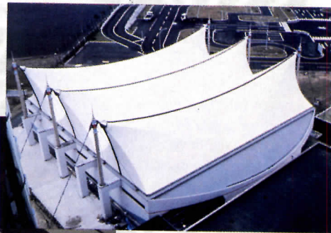
Point-hung tensioned membrane structure at Toyohashi.
