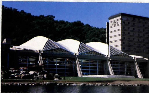
Glass gables are integrated into Sun Palace membrane roof.
