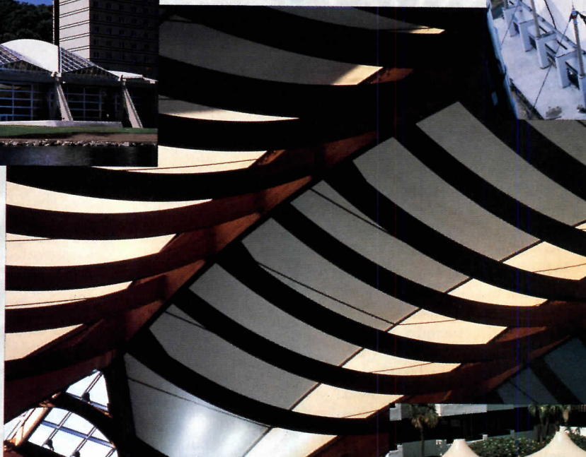
Glue-laminated wood structure supports tensioned membrane roof at Sun Palace swimming facility.
