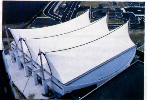
Point-hung tensioned membrane structure at Toyohashi.
