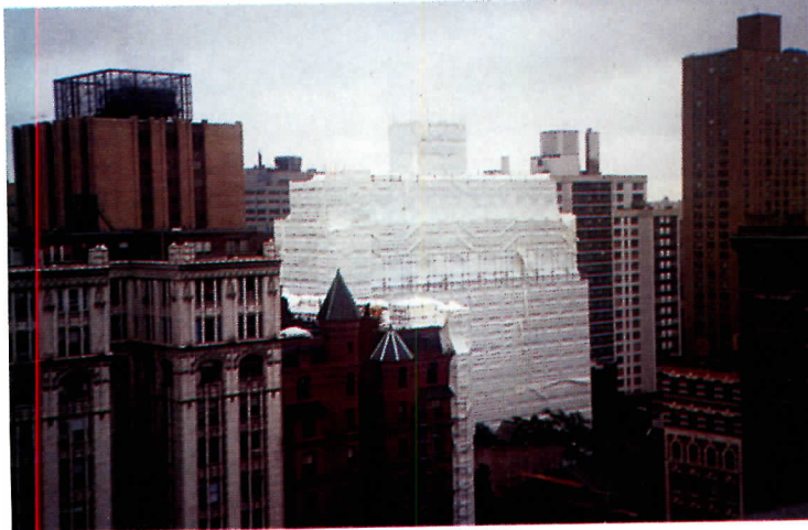
A steampipe explosion in New York City covered an apartment building with asbestos-contaminated mud.
