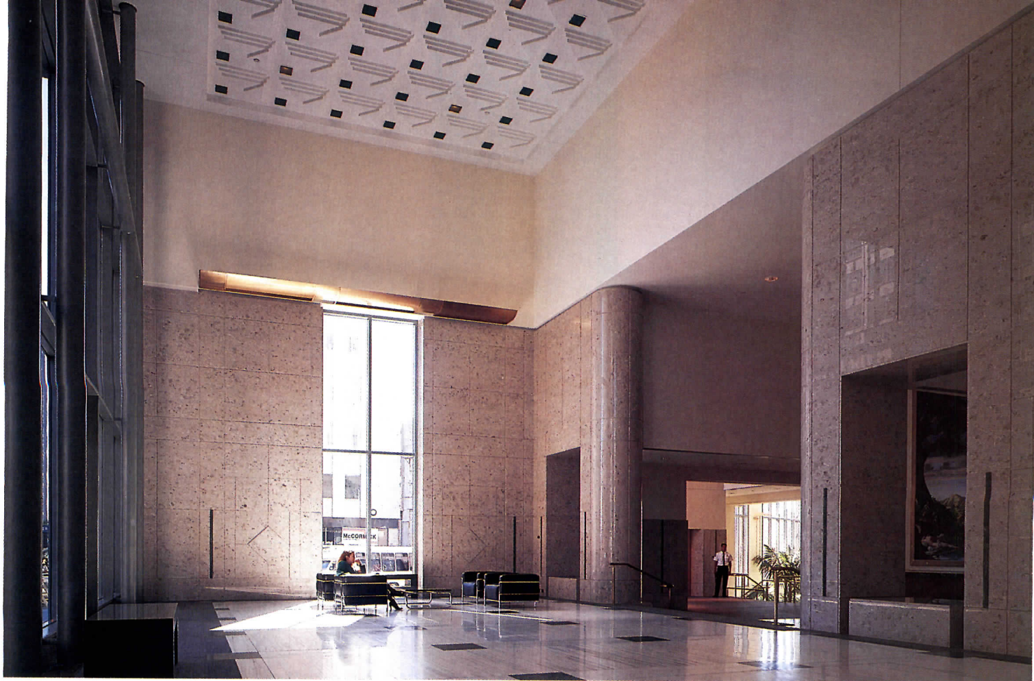
Above: walls of the Wilshire Boulevard lobby are clad in polished Italian marble. Floors finished in striated white statuary marble have green marble accents.
