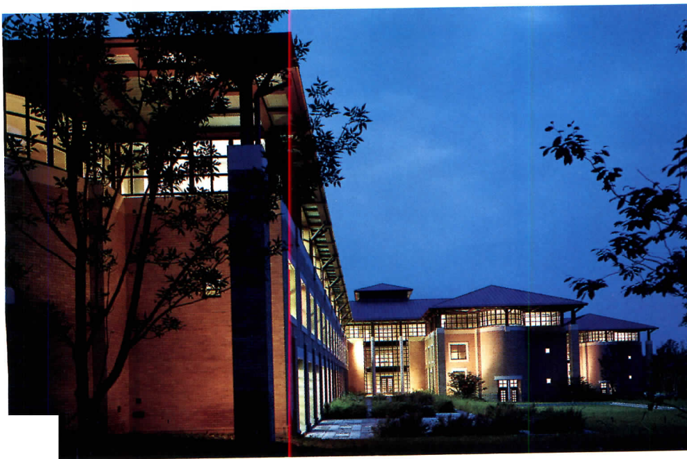
Romance and transparency for a utilitarian structure: Becton Dickinson headquarters; Kallmann, McKinnell & Wood, architects.
