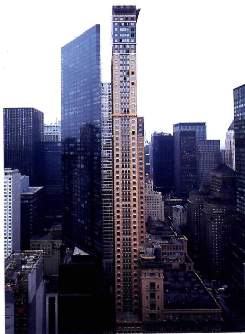
The 50-ft-wide shaft of Carnegie Tower adjoins 16-story Carnegie Hall.
