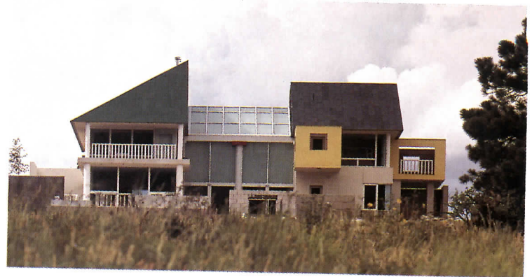
On the south facade, the red entablature atop a giant column helps support the gable of the double-height “glass house.” Yellow boxes are master-bedroom-suite terraces.
