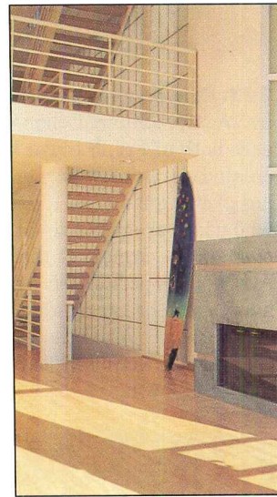
The Fry reveal pattern is continued on the interior walls and around the fireplace.
