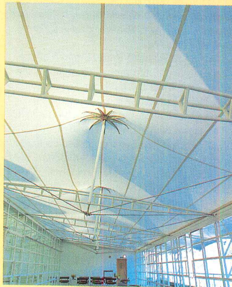
Fabric roofs cover the atrium and a gallery at the Imagination Building.
