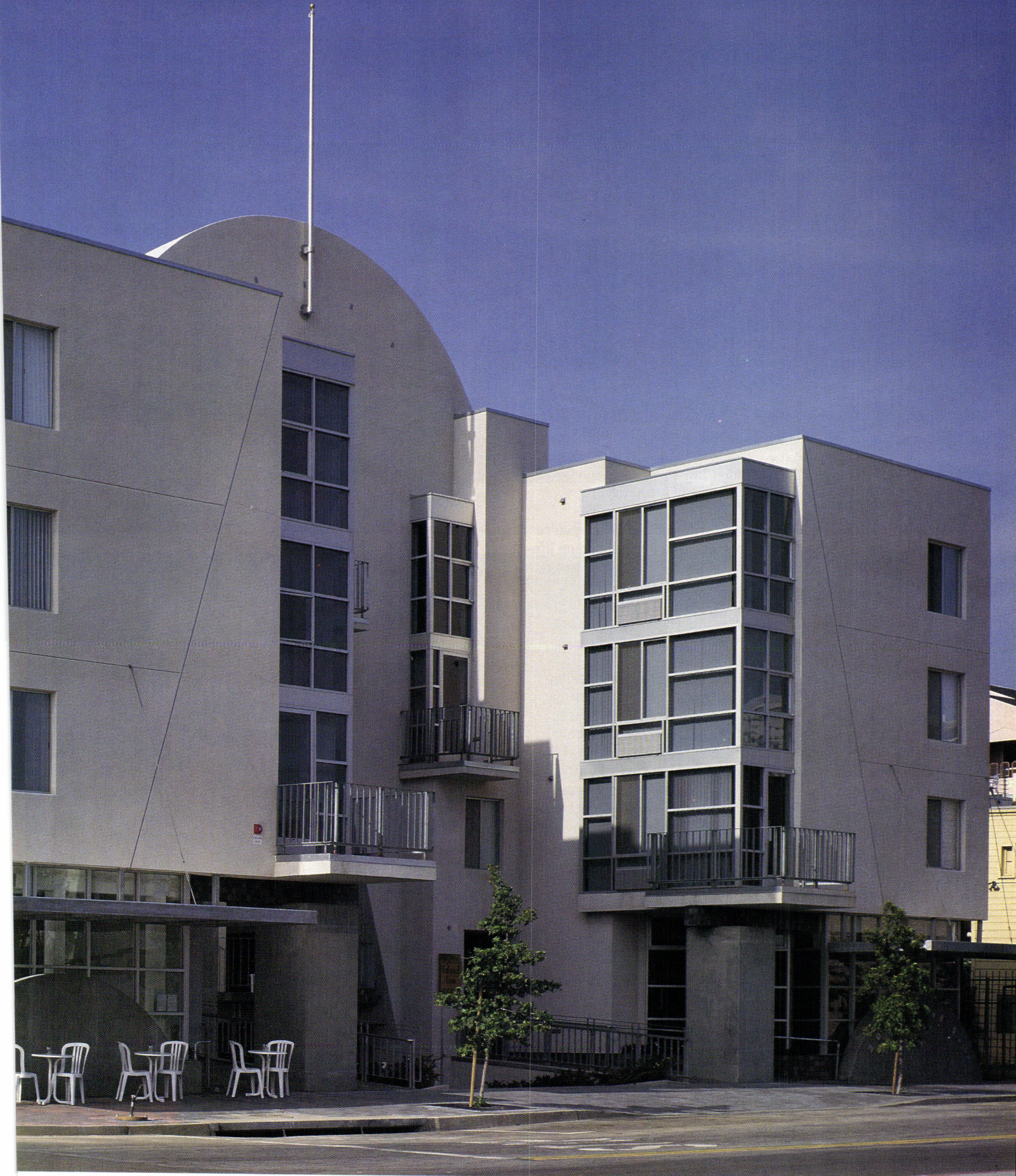
202 Island Inn San Diego, California Rob Wellington Quigley Architect
