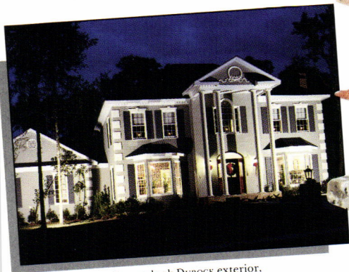
Stucco-look DUROCK exterior, residence, Mobile, AL
