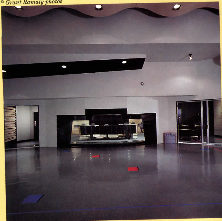
Canted and sloped shapes diffuse sound and prevent unwanted flutter echoes within the main studio.
