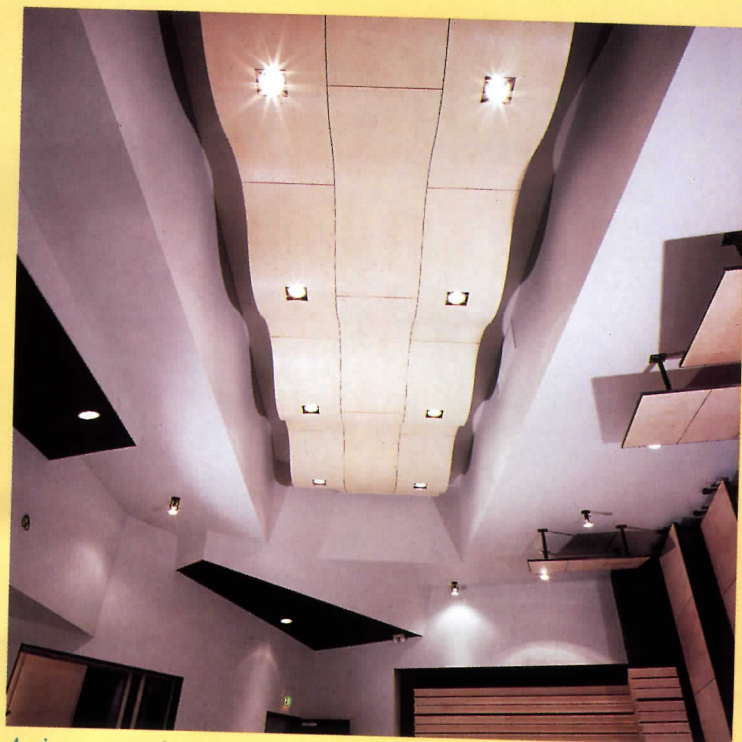
A sine wave of maple plywood breaks up higher frequencies; a layer of fiberglass behind it traps lower frequencies.
