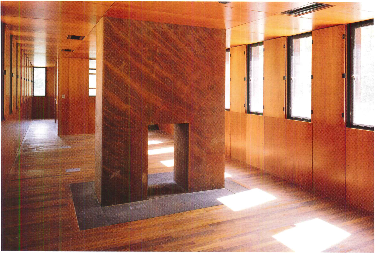
The lower level of the house is 84 feet long from kitchen to bedroom (plans right and opposite). In the center of the 14-foot-wide loft-like space is a steel chimney (above). To accommodate the different expansion rates of steel and wood, interior walls comprise an independent structural frame. Two-foot-wide panels veneered with plantation-grown mahogany are fastened by black painted screws at two-foot intervals to a kiln-dried poplar frame. The bedroom has an Ungers-designed Murphy bed shown closed (top) and open (bottom).
