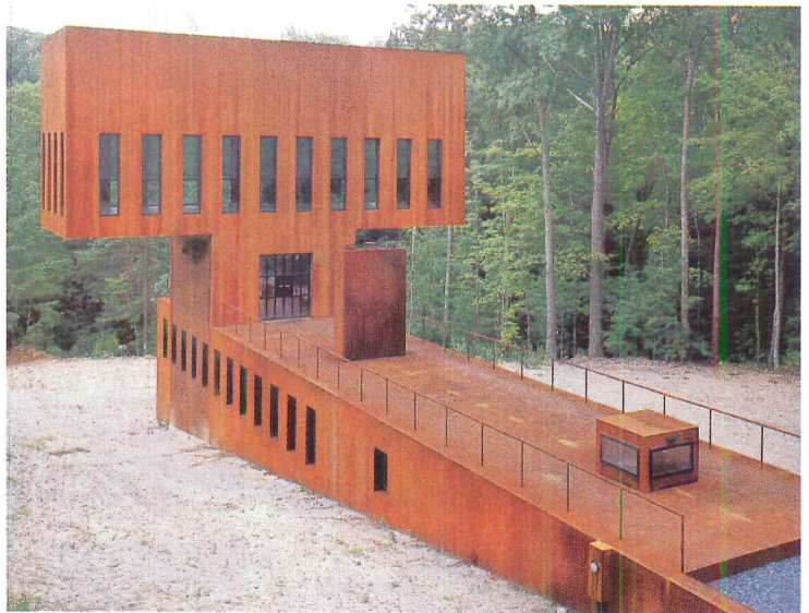
The 1/4-inch-thick steel exterior shell was prefabricated in six parts and then transported to the site, where it was assembled on top of concrete foundations (photo below left). The steel's nickel and chromium finish has oxidized to a vibrant rust color.
