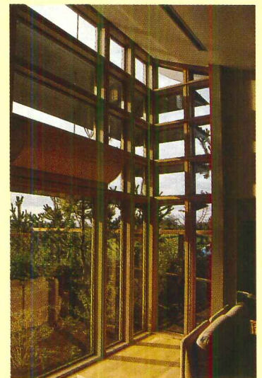
Top: Detail of galvanized-steel fins that bounce summer light up while permitting direct passage of winter light. The orientation virtually keeps out direct sunlight in summer. The concrete column system is separated from the body of the house and is not structural. Bottom: corner at living room.
