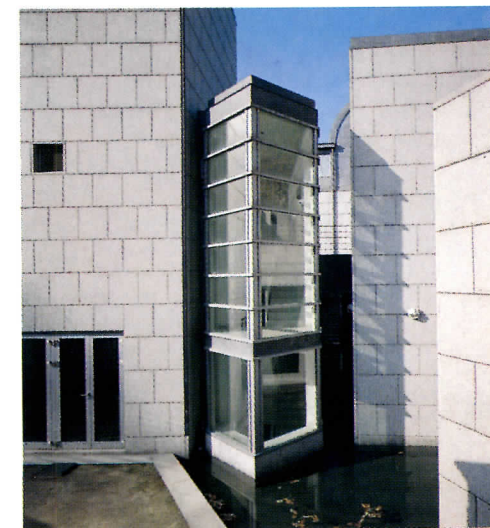
The museum sits on a rough-hewn granite base, its walls clad with smooth granite panels (top and bottom). The annex and compound wall are made of contrasting concrete brick (middle). Elements meeting the sky are covered with lead-coated copper (opposite).
