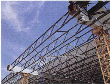
90' Vulcraft steel joists.
