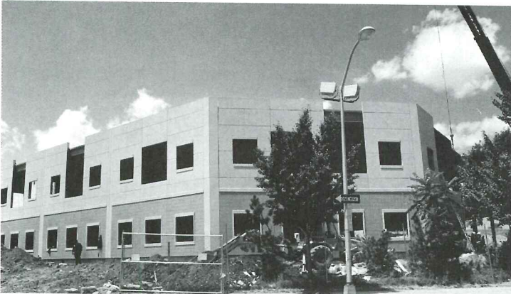
175. Lightweight precast. A new exterior cladding, stud-backed Slenderwall panels are said to provide the decorative and weatherproofing performance of conventional precast panels at a significant weight savings. Architect Ken Rubsamen of Rothe/Johnson Corporation used 1/2-in.-thick tiles to match a new Technology Center with other buildings at Essex College in New Jersey. The panel has 2-in. of reinforced precast, with steel studs cast into the concrete and held by stainless-steel Nelson anchors. System is said to save on footings, framing, and heating costs. Finish options include face brick, clay tile, and exposed aggregate. 800/364-3981. Smith/Midland, Midland, Va.
