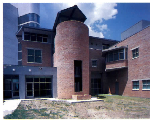
The $3-million building opened in September at a cost of about $107 per sq ft. The first two floors of the building are a concrete-frame structure, while the third floor is framed in steel.
