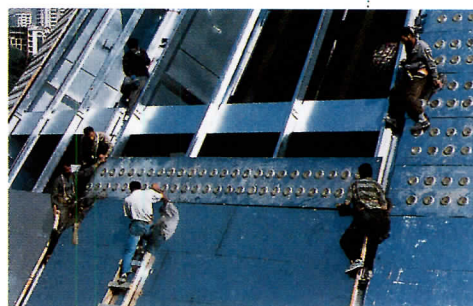
The main facade of the 250,000-square-foot International Conference Center in Teheran (above). Local laborers work on the dome, whose panels were fitted with 40,000 glass cylinders (left).
