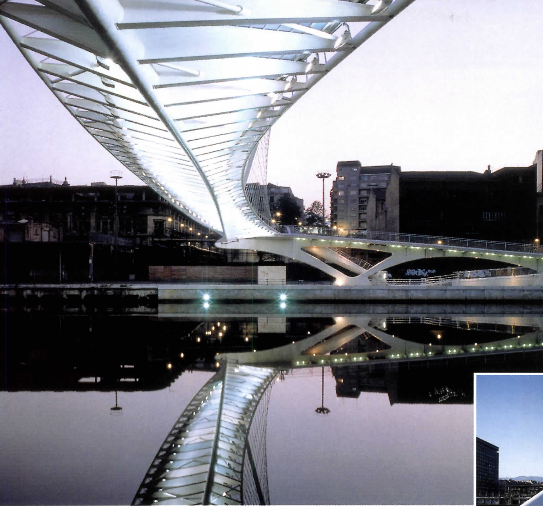
THE CAMPO-VOLANTIN BRIDGE , in Bilbao, Spain (1990–97), spanning 232 feet, acquires a visual dynamism from its inclined parabolic arch structure. Its curving path and translucent paving become especially dramatic when illuminated from below at night.
