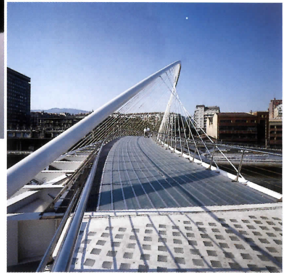
THE CAMPO-VOLANTIN BRIDGE , in Bilbao, Spain (1990–97), spanning 232 feet, acquires a visual dynamism from its inclined parabolic arch structure. Its curving path and translucent paving become especially dramatic when illuminated from below at night.
