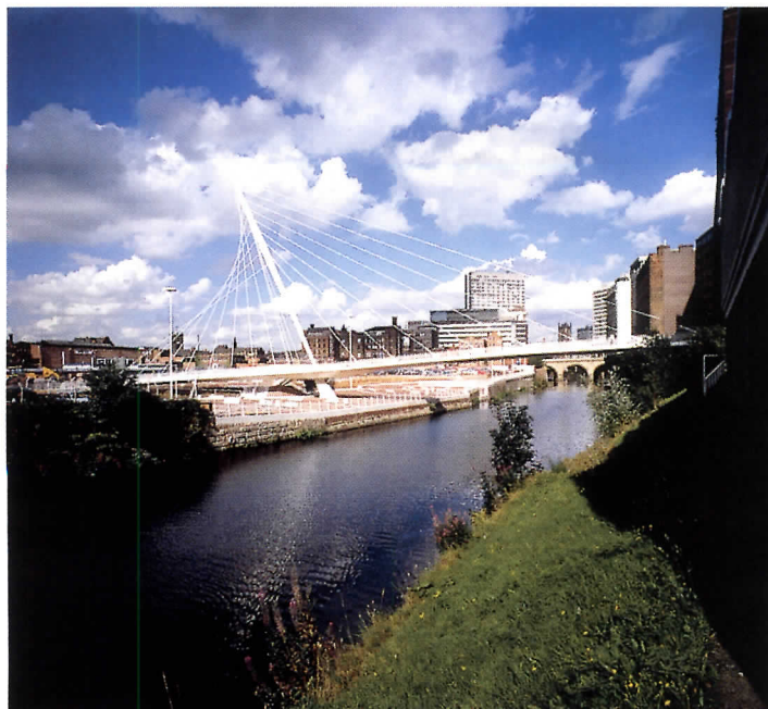
THE TRINITY FOOTBRIDGE in Salford, England (1993–95), achieves extraordinary balance and a quality of formal essence. A 135-foot-long pylon, inclined at a 30-degree angle, supports the span.
