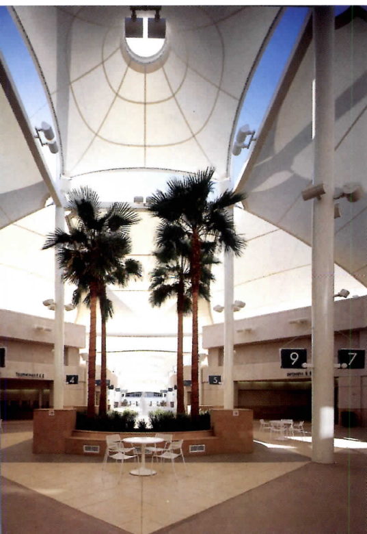
Teflon-coated fiberglass canopies help create shaded outdoor rooms at the new 11-
