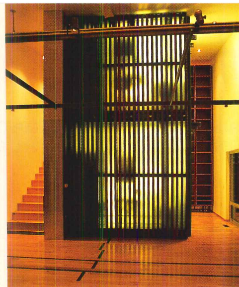
Bathroom walls of polycarbonate divide and define spaces in both houses. The degree of opacity at 216 Alabama (left) or the addition of color at 1603 Random Road (right) are used to vary the effects of light and shadow.
