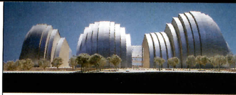
Stainless-steel walls will curve up the back of the theaters (top), which share a lobby.
