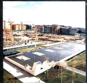
The architects won over neighbors of the mortuary by slipping the 345,000-square-foot building under a large reflecting pool.
