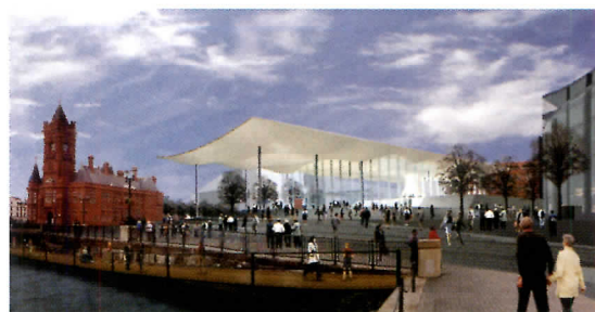
The Welsh Assembly headquarters, designed by Rogers.
