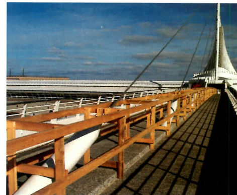
A temporary railing at the Milwaukee Art Museum.
