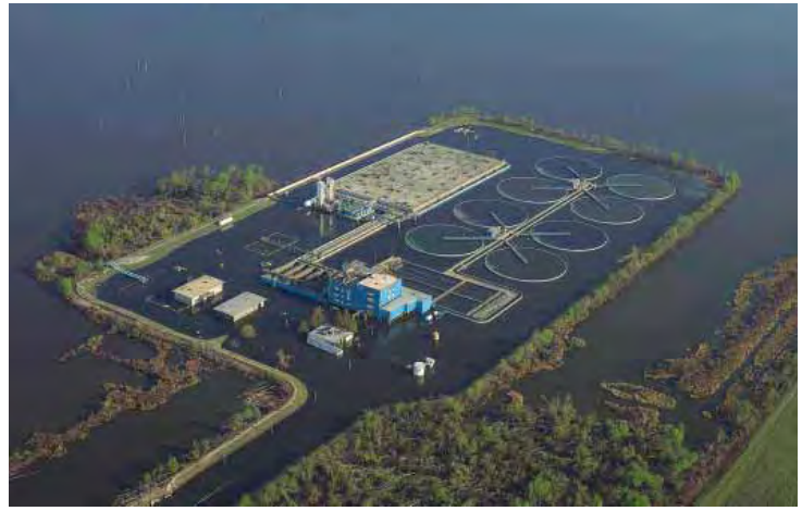
The floodwaters inundated many wastewater treatment plants in and around New Orleans, making the safeguarding of water quality even more difficult.
