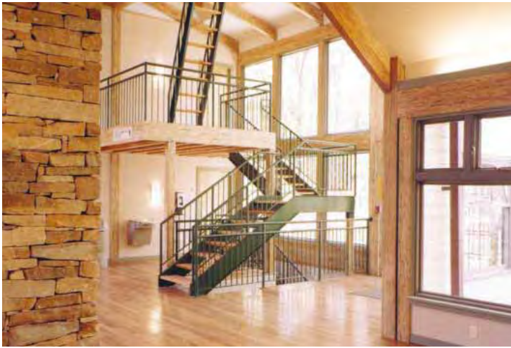
Floors of locally sourced white oak work sustainably and efficiently with a geothermal radiant heat system at the Girl Scouts' Eberly Family Learning Center in West Virginia.
