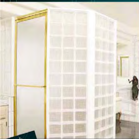
45-degree corner caps were used to connect Hy-Lite panels to form this neo-angle shower. Flat caps were used to finish off the top and sides of the doorway, while a flat cap and mounting channel were used to attach the panels to the curb and wall.
