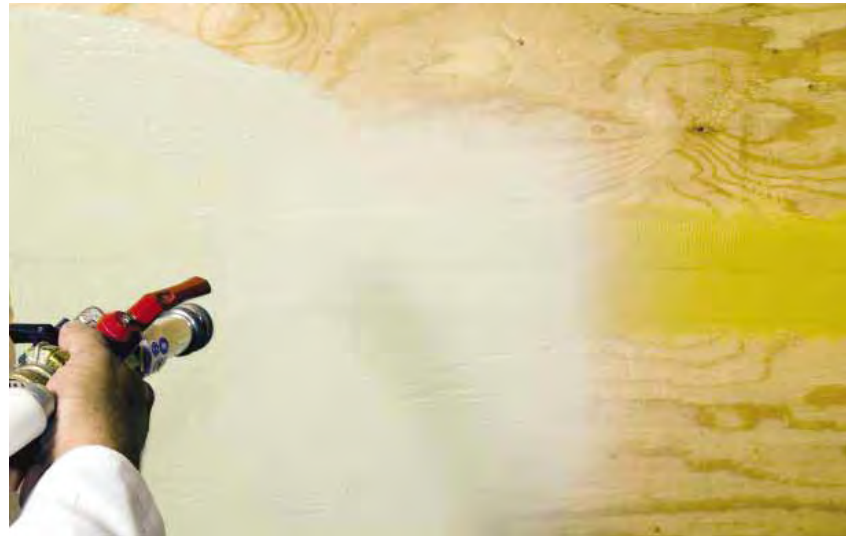
Figure 1b: Fluid applied air/moisture barrier applied to sheathing by spray application.
