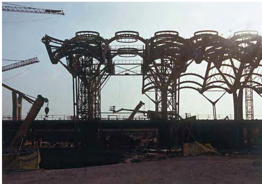
At Terminal 4 at Barajas Airport in Madrid (above), designed by Richard Rogers and Estudio Lamela, the same long-span roof module was applied consistently to multiple segments.
