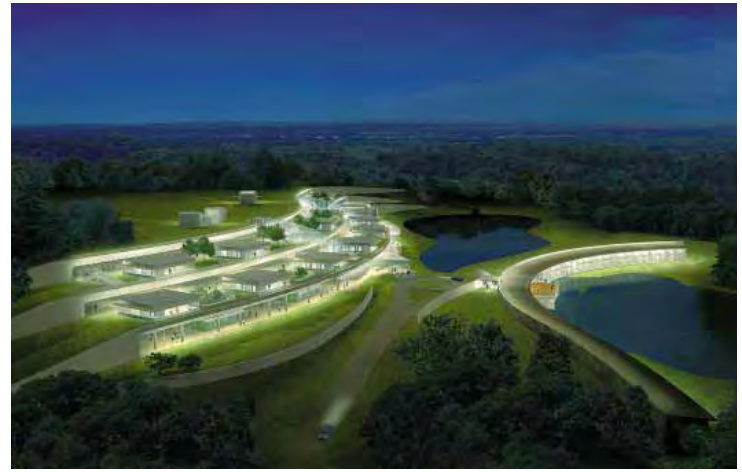
The new, 610,000-square-foot campus is being built into a bluff.
