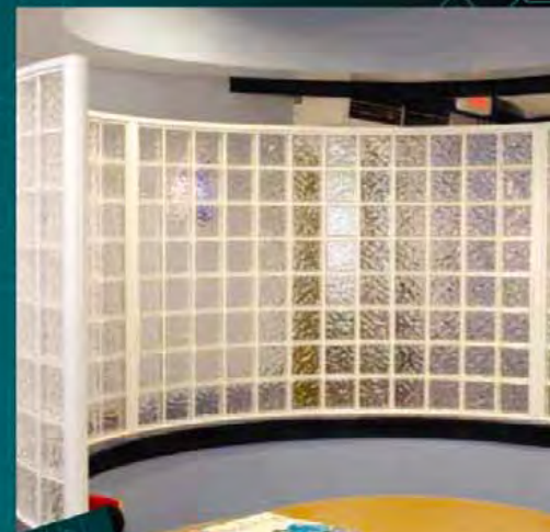
Round caps finished off the ends of this radius wall perfectly. Aluminum mullins were used to connect the three radius walls together, while a flat cap mounted the units to the top of the curved wall.
