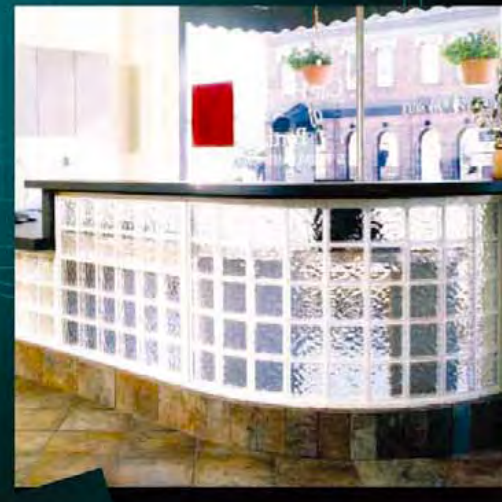
Aluminum mullins were used to connect these flat panels and radius walls together. A flat cap and mounting channel were used to mount the units to the base and the walls. Flat caps were also used to connect the desktop to the top of the panels.
