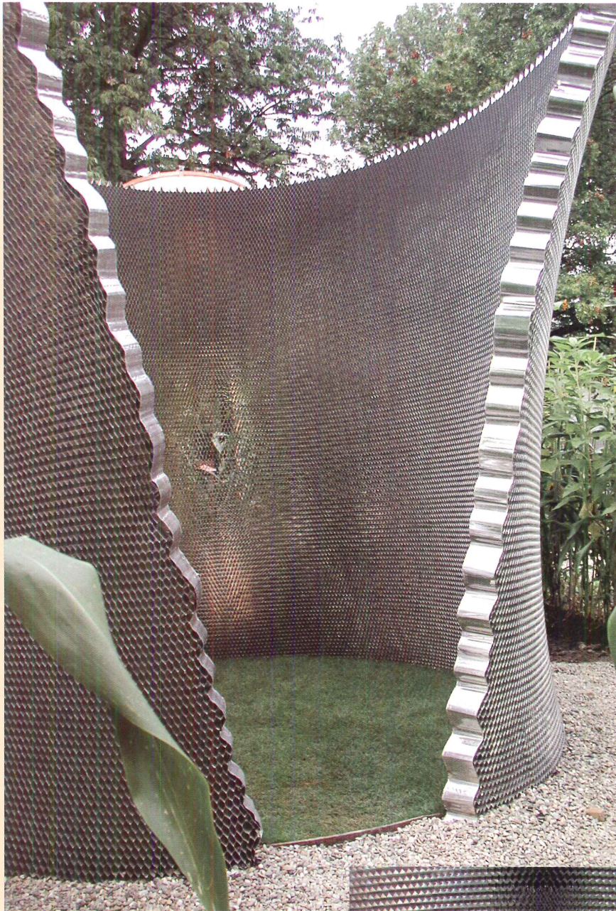
Sharon McHugh and John Nastasi Architects built the Cornel West Pavilion in 2004 with Nastasi's graduate students at Stevens. This temporary, self-supporting structure on the campus of Princeton University is made from a honeycomb metal mesh used in the aerospace industry. Its geometry was derived from a digital study of the material's structural properties.
