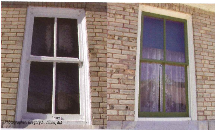
Window before and after restoration by SmithGroup at Old Mackinac Point Light Station
