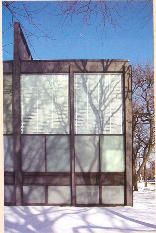
At least five full-size mock-ups (above) were produced to test several glazing options and the blind replacements. Studies of solar radiation transmission show the difference between laminated glass units (top left) and single sandblasted panes (left).
