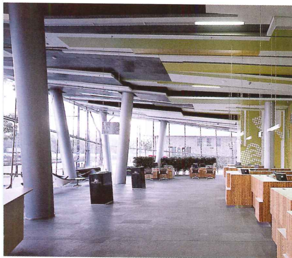
ING offers 270,000 square feet of space on seven floors with plans that provide plenty of daylight in offices and spaces such as the banking hall (left).
