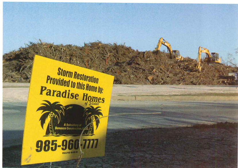
Orange waterlines are sometimes the only clue to the devastation inside homes and buildings. Canal Boulevard, near City Park, has been turned into a giant trash dump.
