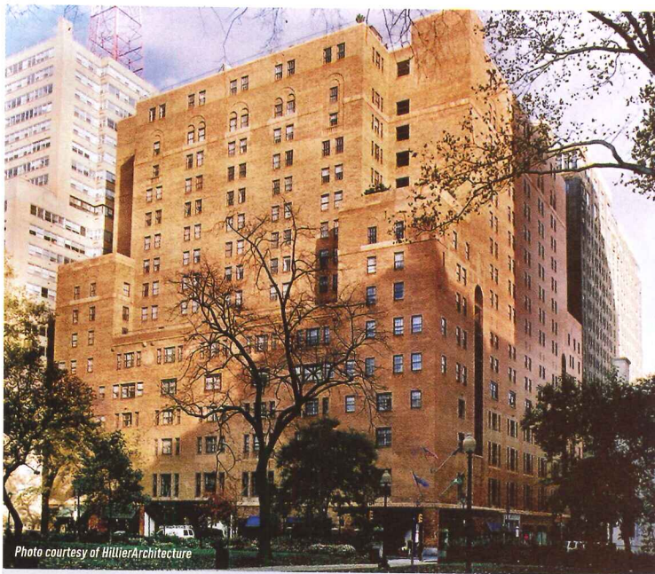
Photo courtesy of HillierArchitecture Parc Rittenhouse, Philadelphia, PA, before conversion by HillierArchitecture
