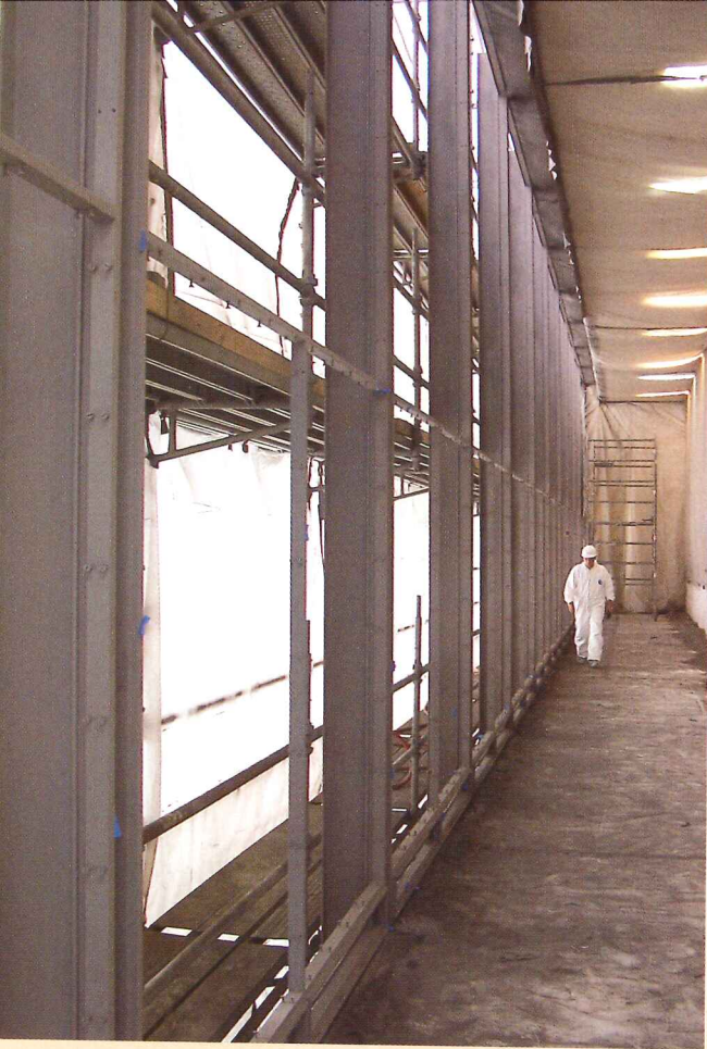
New frames and tops are in place, awaiting installation of the glass (above). The difference between the original detail (top right) and the new one (right) is very subtle.
