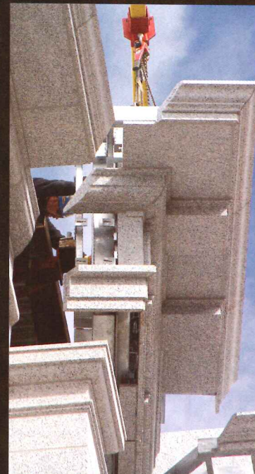
Granite Entablature Panel UT State Capitol Expansion
