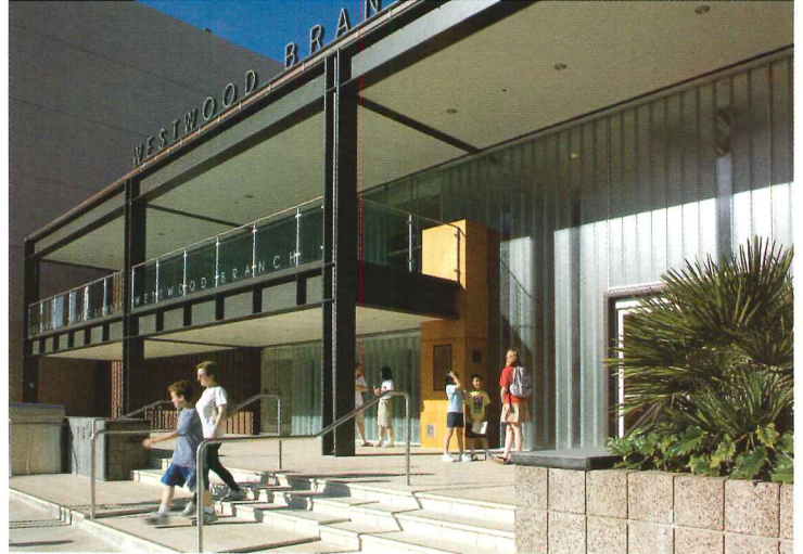
Channel glass in the facade of Steven Ehrlich Architects' Westwood Branch, in L.A., controls light levels and blocks views of parking lots across the street.
