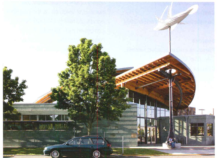
A kinetic steel boat sculpture sails above the roofline of Carlson Architects' Beacon Hill Branch in Seattle. Each new library there features public art.
