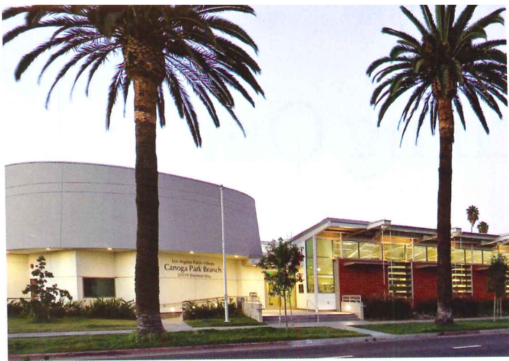
The bold facade of Carde Ten Architect's Canoga Park branch, in L.A., provides a welcome counterpoint to nearby burger joints, strip malls, and parking lots.
