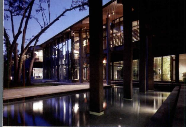
Helfand Architecture Automated Trading Desk Technology Campus, Mount Pleasant, S.C., 2002
