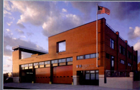
Karahan & Associates Combined Fire and Emergency Medical Service Station, Rockaway, N.Y., 2004
