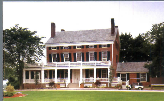
Page Ayres Cowley, Architects La Tourette Golf Club House restoration, Staten Island, N.Y., 2003
