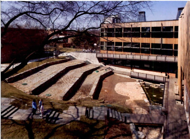
The plants in the terraces of Sidwell's subsurface-flow constructed wetland (left) are expected to grow in over the summer. Subsurface wetlands (above) control odors and environmental hazards by keeping water underground.
