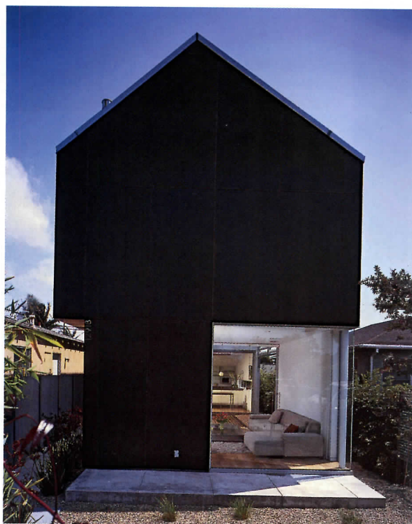
The living room window (above two) allows views to the rear of the house.
