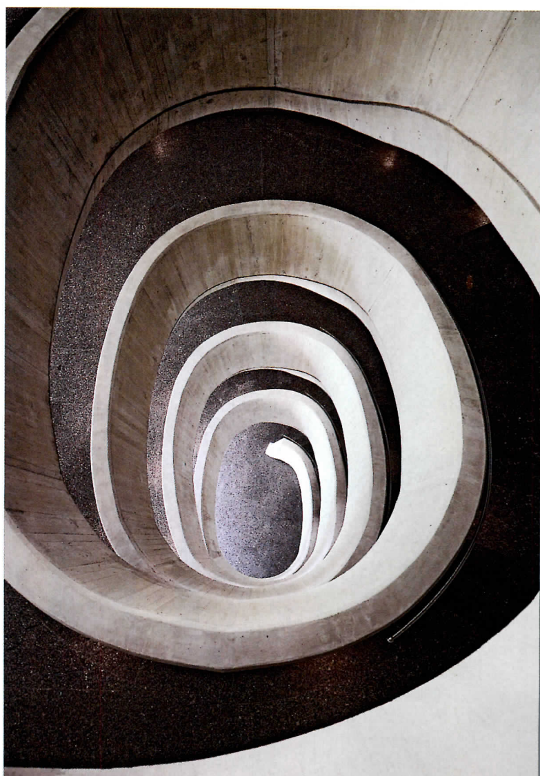
Calatrava's structural and formal exuberance shapes virtually every aspect of the building, from the restaurant's steel members (left) to a spiral stair (right).
