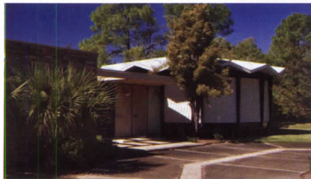
The Cohen residence, shortly before demolition.
